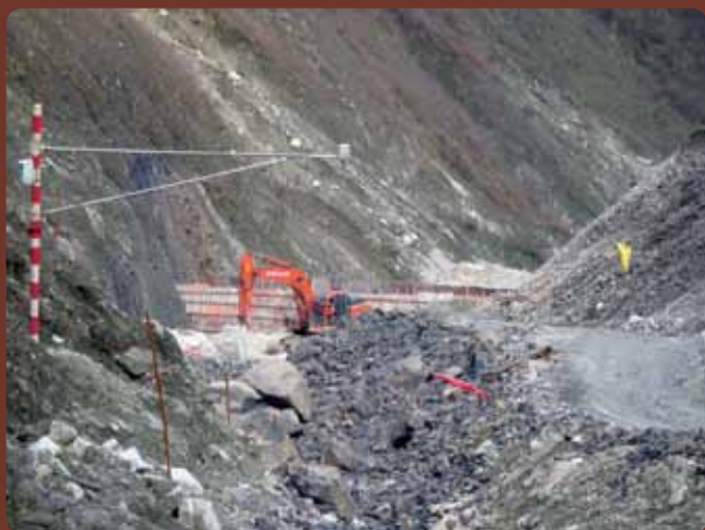
Figure 28: Alarm system installed in the headwaters of Niujuangou gully
