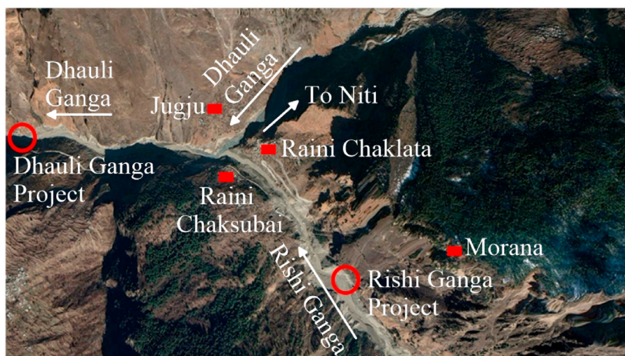
Fig. 6. The affected hydropower projects and villages after calamity (Google Earth, 2021).
