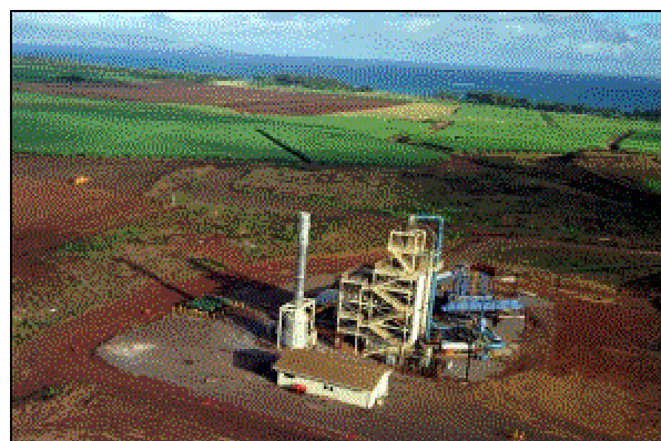
Residues from crops can be gasified and combusted to provide heat and power. (Photo courtesy Warren Gretz and NREL.).
