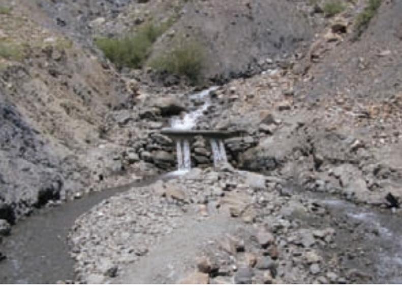
Figure 6: Nirwalu – an indigenous system of water distribution in Mulkhow
