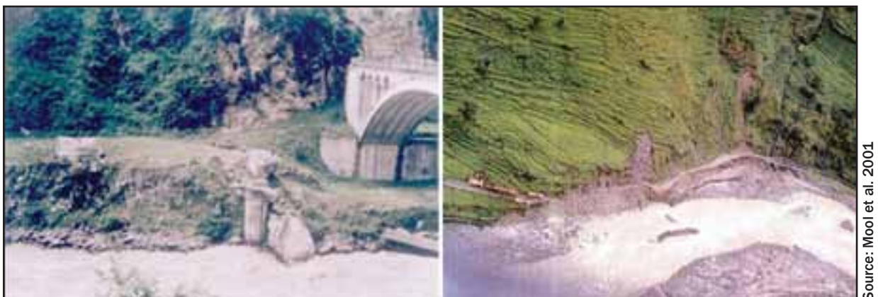
Figure 20: Remnants of a bridge pier (left) on the Arniko Highway and a section of the highway destroyed by the 1981 Zhanzangbo GLOF
