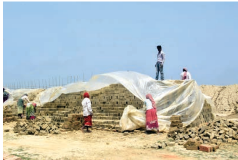
PROTECTING STACKED GREEN BRICKS FROM THE RAIN IN PROVINCE 1
