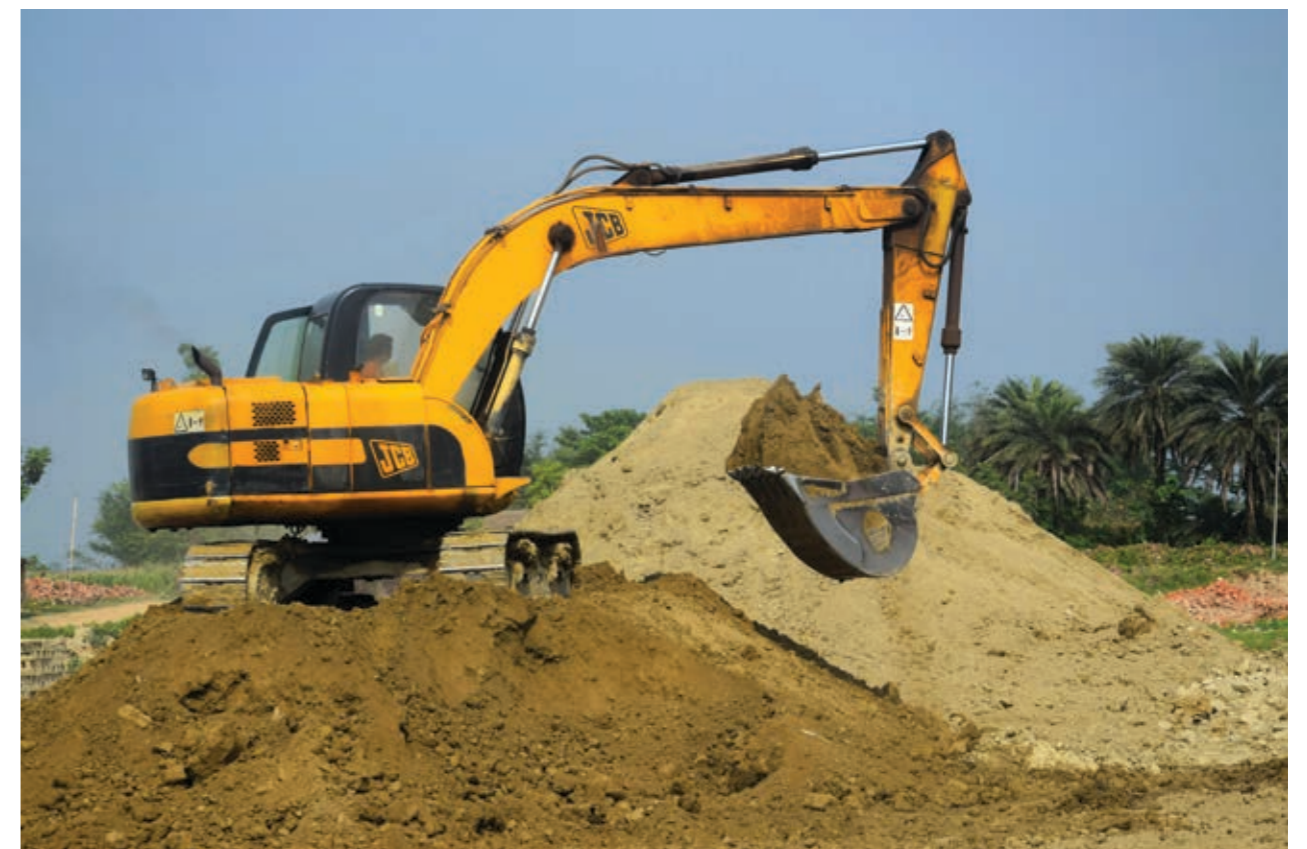
AN EXCAVATOR IN RUPANDEHI ARRANGES SOIL FOR MOULDING
