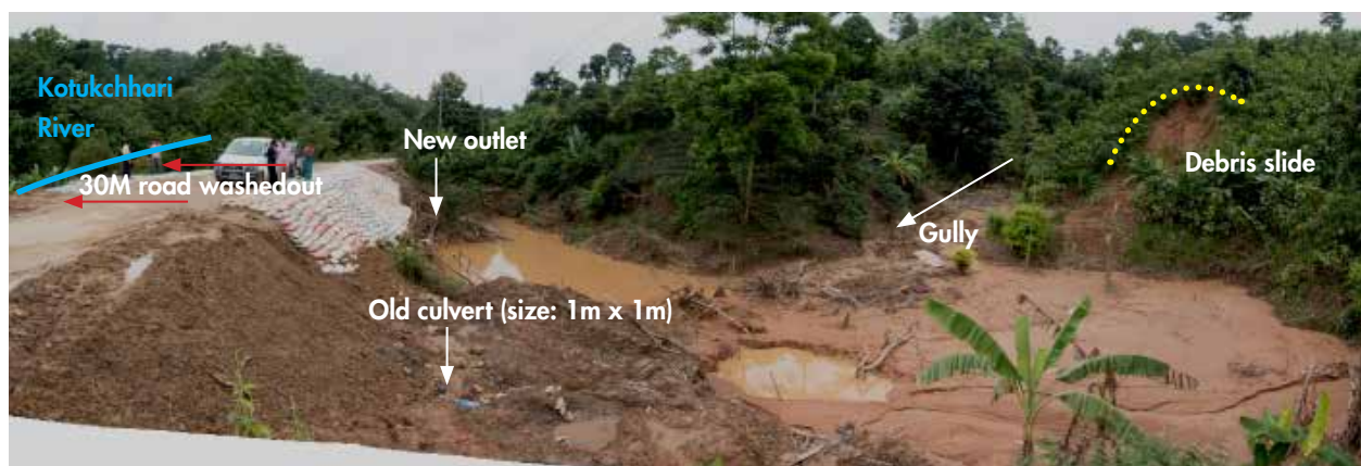
Figure 17: Drainage blockage outburst at Montola Kijing (Rangamati-Khagrachhari Road) (Note: New outlet made of about 60 cm diameter is not large enough in case trees and debris block the culvert.)
