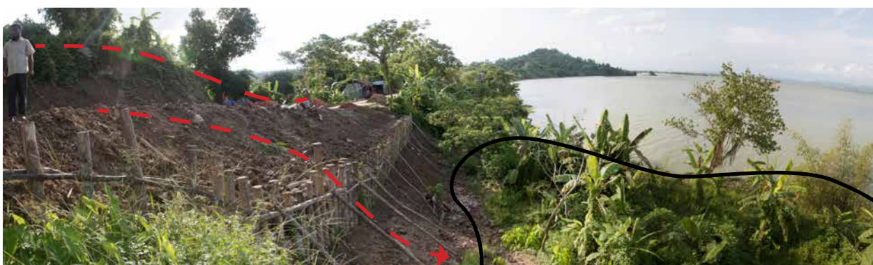
Figure 19: Subsidence and debris flow at Banabhante (Rangamati-Kaptai Dam Road)
