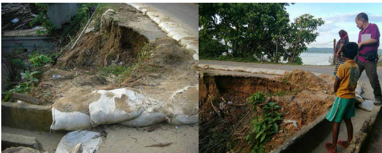
Figure 15: Road side slope failure due to under-capacity road side drainage at Risermok
