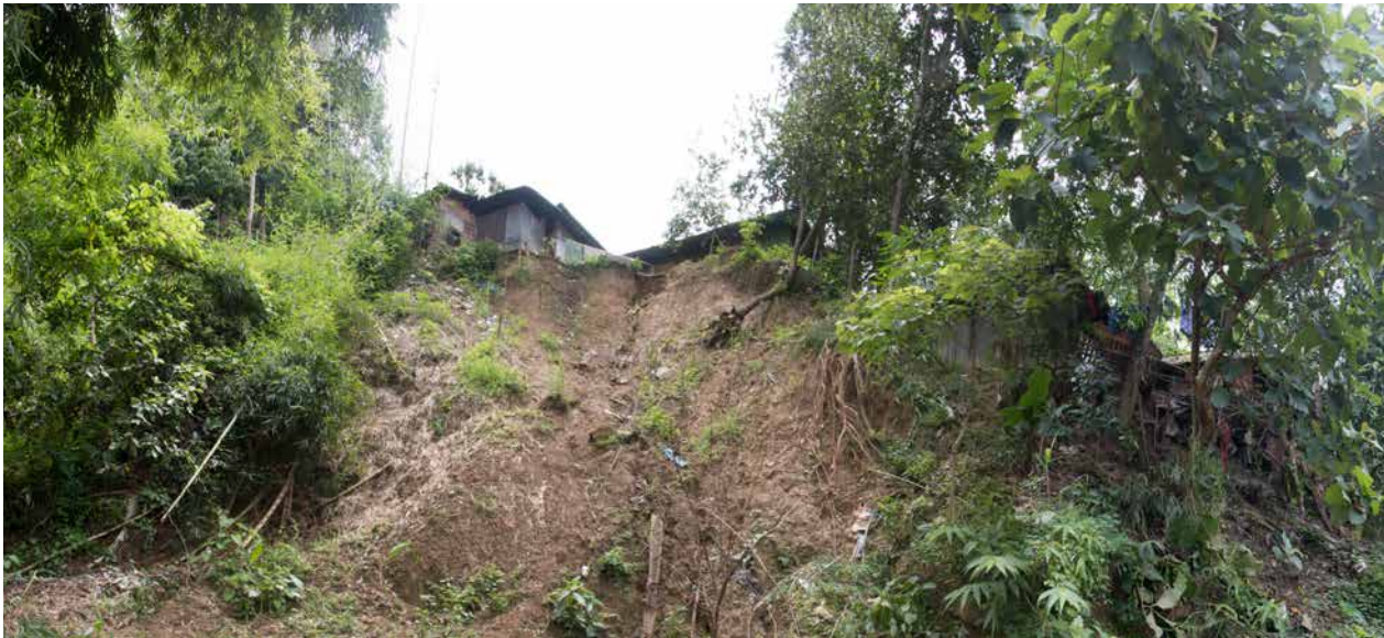
Figure 9: Catchment gully head failure at Ghagra Bazar (50 m south of road junction of Rangamati-Kaptai Road)
