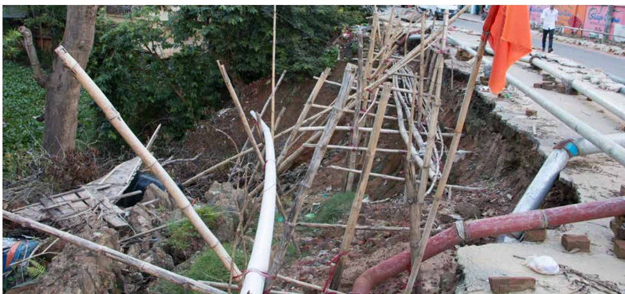
Figure 14: Road side slope failure due to water supply leakage
