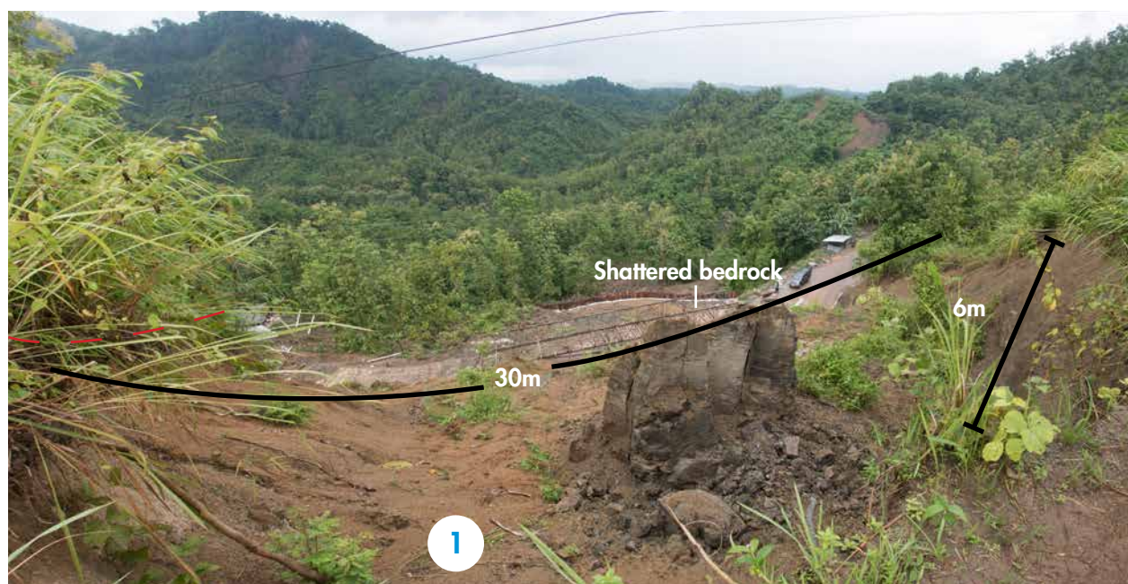
Figure 7: Hill slope failure at Sapchari-Salbagan Bailey bridge site
