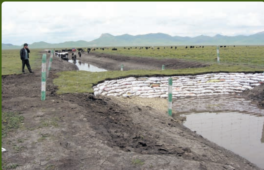
Figure 21: Typical drain-blocking site in the Zoige Peatlands, China
