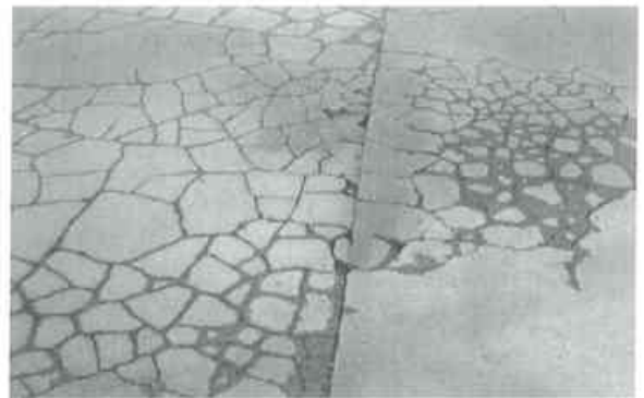
Figure 2.1: Minor cracks on road surface
