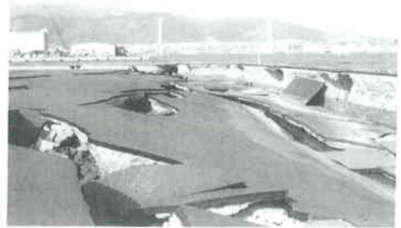
Figure 2.3: Road structure collapses
