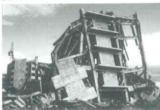
Figure 5.3: A reinforced concrete collapsed building (Tadjikistan, 1985)
