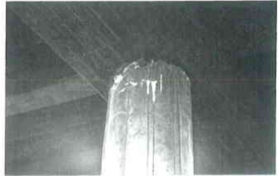
Figure 2.6: Minor cracks on a pillar
