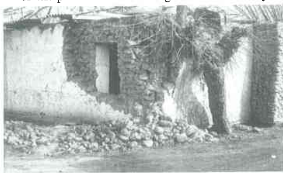
Figure 5.2: A collapsed mud-brick house (Armenia, 1988)
