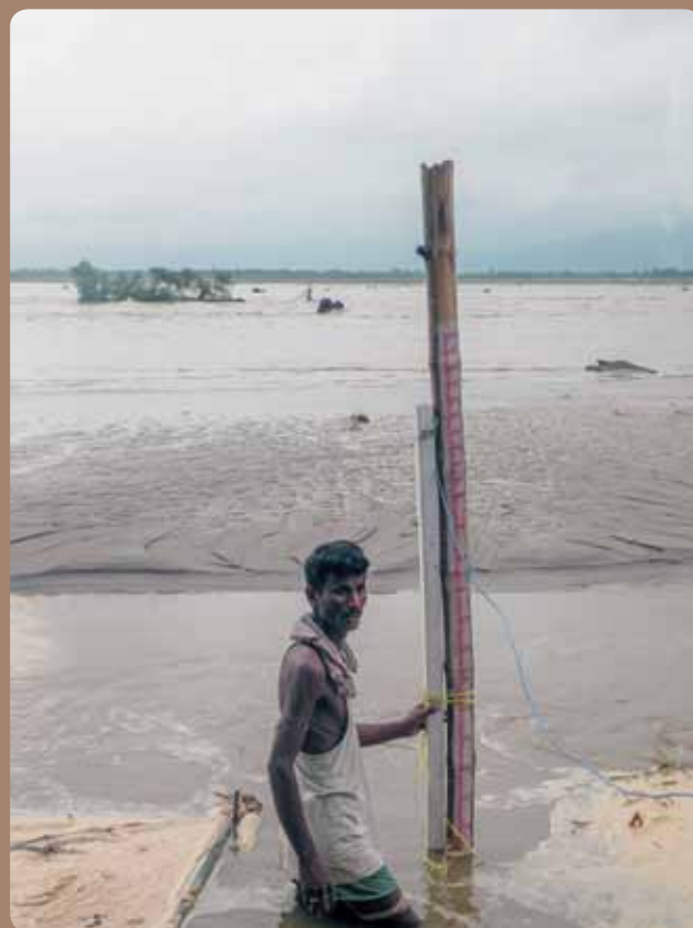
Figure 11: Installation of a flood gauge at Barmaba village
