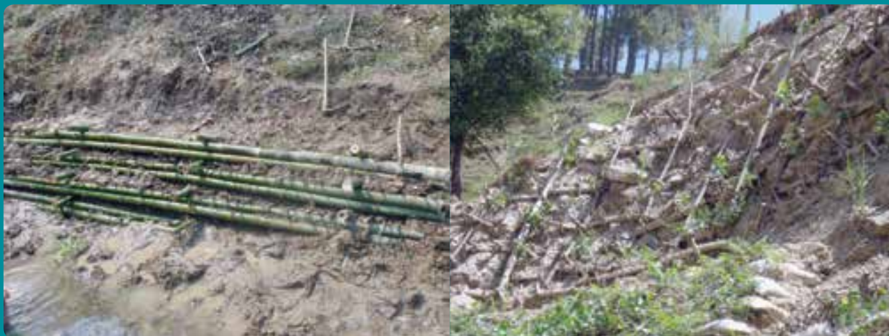
Figure 16: Newly constructed live crib wall made of bamboo (left) and live crib wall on a slope (right)
