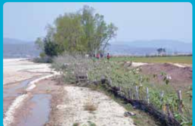
Figure 21: Wattle fence used for river bank protection
