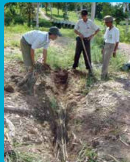
Figure 18: Installing live fascine
