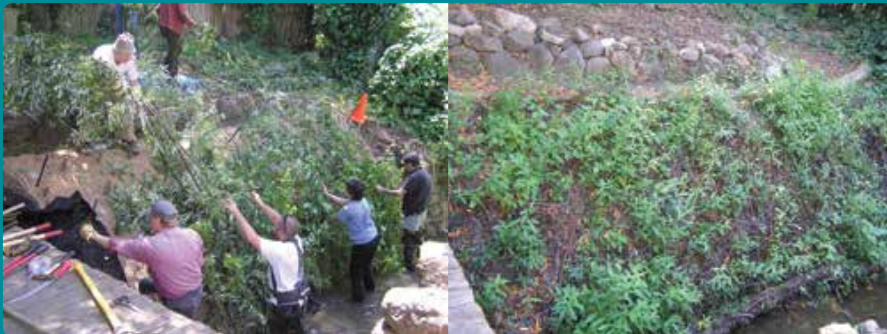
Figure 12: Installing brush mattress
