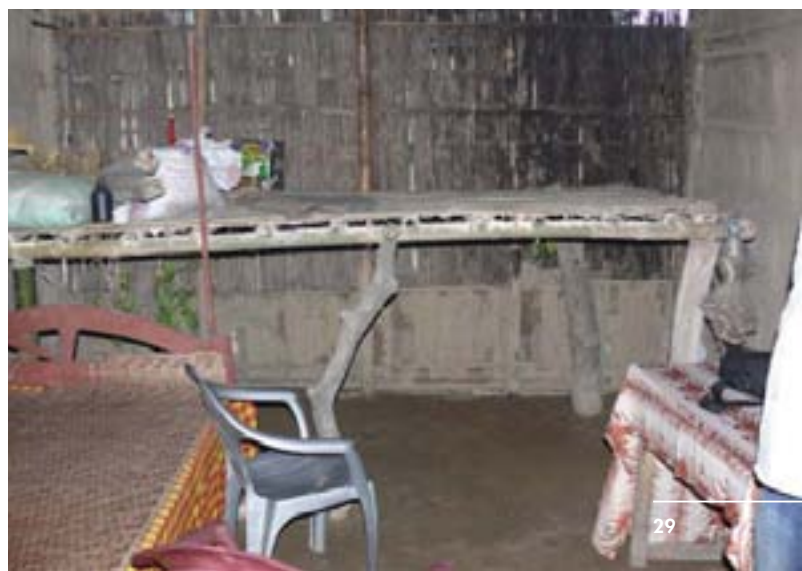
Figure 15: A raised platform inside a house gives shelter during floods: adaptation practice of non-Mishing communities in Majgaon
