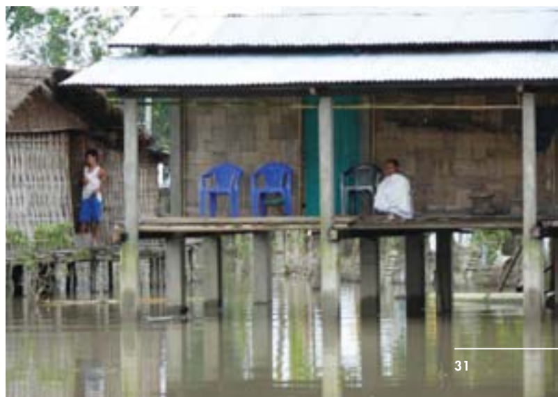
Figure 16: A 'chang ghar' (stilt house) of the Mishing community in Matmora – a classic example of adaptation to floods
