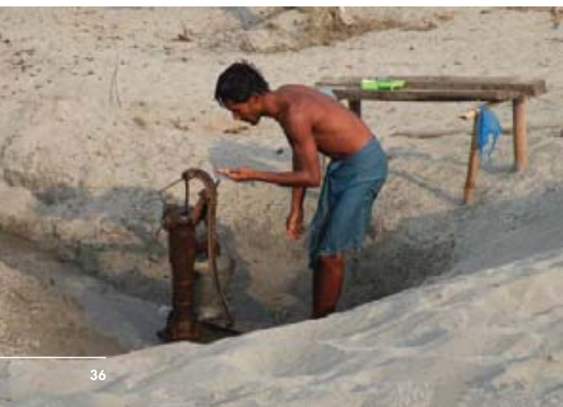
Figure 20: Entombed water: people digging out tube wells buried under layers of sand and reusing the same as seen in Opar Khamon village, Matmora
