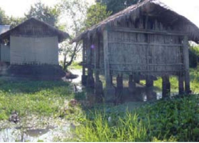
Figure 17: A traditional Assamese house built on an elevated platform (left); the separate granary built on stilts (right) has provision for a living space during floods.
