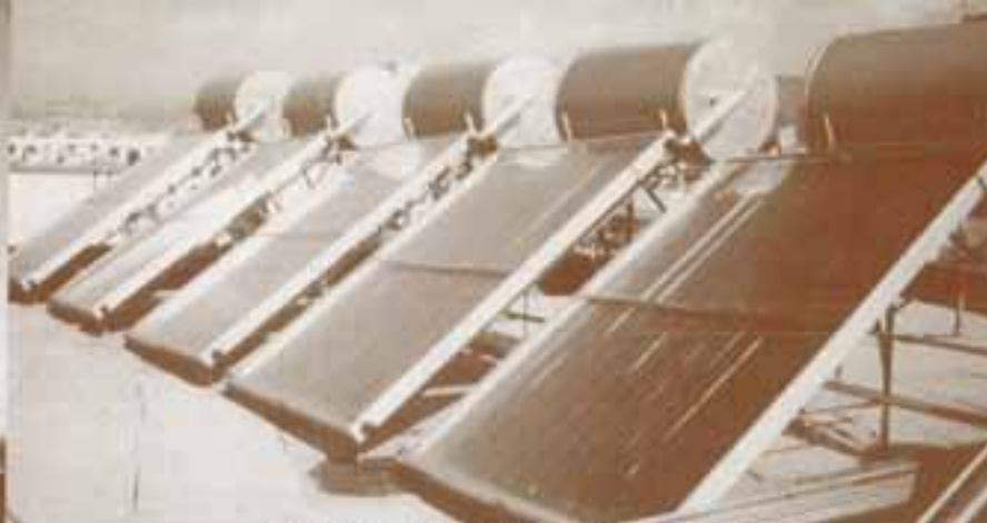
Solar water heaters on the roof of an apartment building in Kunming, P. R. China
