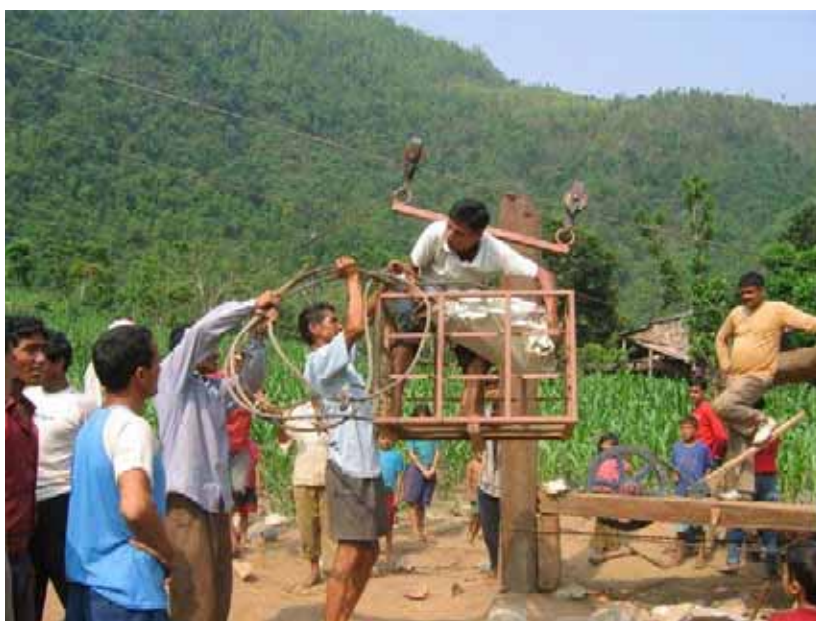
A gravity ropeway under construction using local labour and materials
