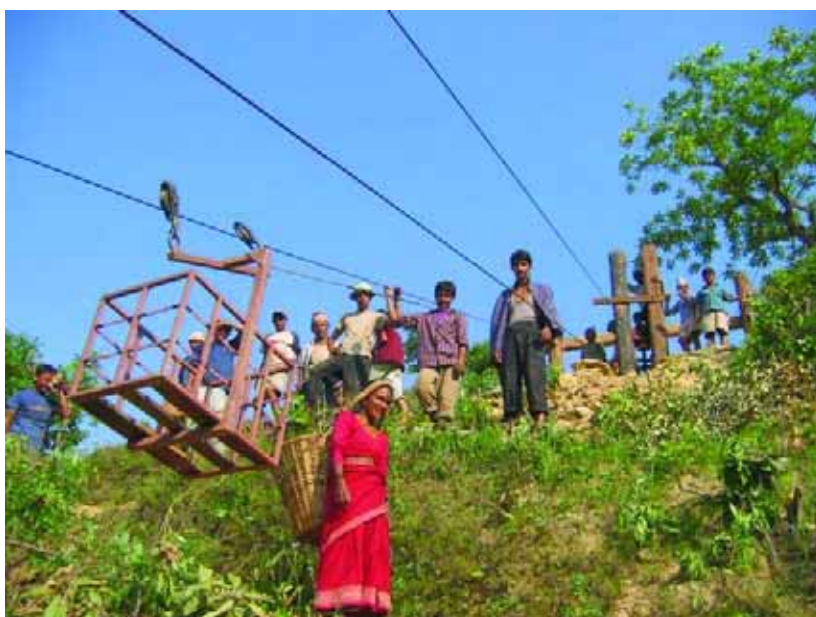
Testing the newly constructed gravity ropeway in Janagaun, Dhading District, Nepal
