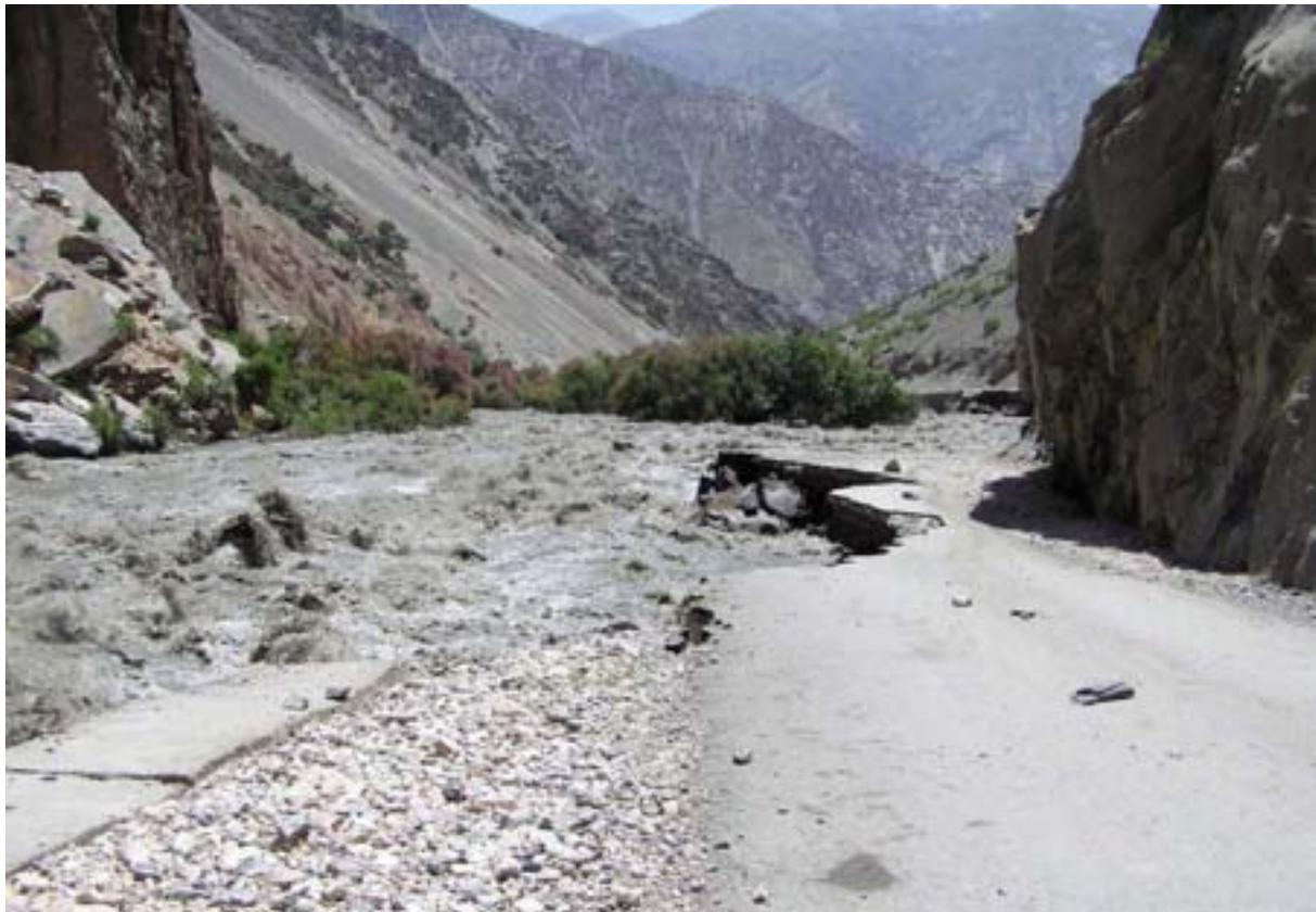
Figure 6: Damage to highway by a flash flood in July 2005 in Garam Chasma, Chitral, Pakistan
