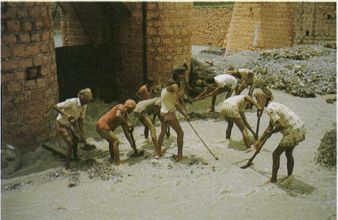
The urban water supply of Dehradun during the monsoon months is maintained at heavy cost because of the constant need to divert the debris away from the main intake point. Any delay in doing so will "choke" the whole water supply system causing heavy losses.
