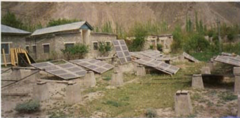
Plight of solar photovoltaic electrification scheme at northern areas of Pakistan due to lack of maintainance.
