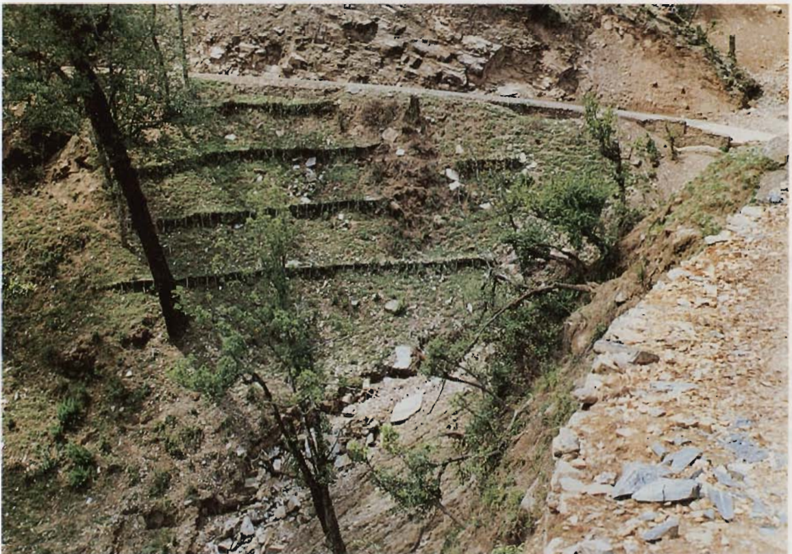
Plate 23: A vs road slope is protected by mini toewalls out of wood to retain the dumped surplus material and by planting grass bunches with fast growing and deep rooting properties).
