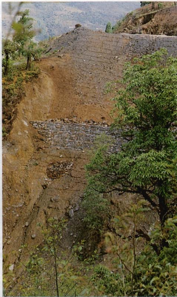
Plate 24 Vs slope protection after slide with 2 checkdams (only the upper one is visible) and mini terraces with plantation just after completion of work).
