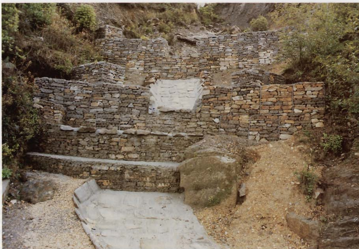
Plate 19: Inlet protection of a gully by two checkdams with channeled water flow and stone slab covered checkdam crowns and steps.
