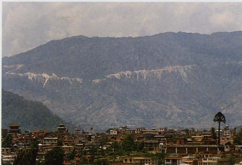
Plate 13: This road has been completely hewn into the slope and the whole excavation material thrown over the vs road edge thus devastating all the vegetation below. Such huge scars can hardly be healed by erosion protection measures and will become bigger and bigger during the monsoon seasons and finally leave no other way than to re-align and reconstruct the road.
