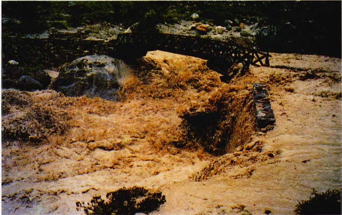
Plate 17 A small glacial lake outburst flood disrupting a bridge on the Dudh Kosi river, Central Nepal, July 1984 (photograph by J. Desloges).
