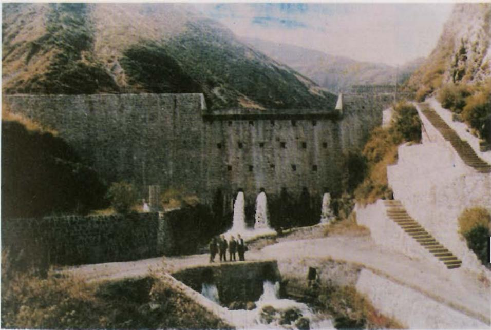
Plate 6: An Arched - Foundation - Masonry - Sifter Type Checkdam, 23m high, in Babuli Ravine, Jinchuan County, Sichuan
