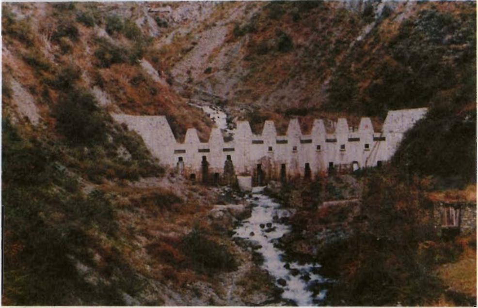
Plate 7: A Sawtooth-Type Checkdam, 10m High in the Babuli Ravine, Jichuan County, Sichuan
