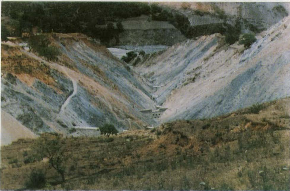
Plate 4: Stepped Checkdams to Control Landslides and Debris Flow in the Daqing Ravine of Daxueshan, Yongbi County, Yunnan - Li Deji
