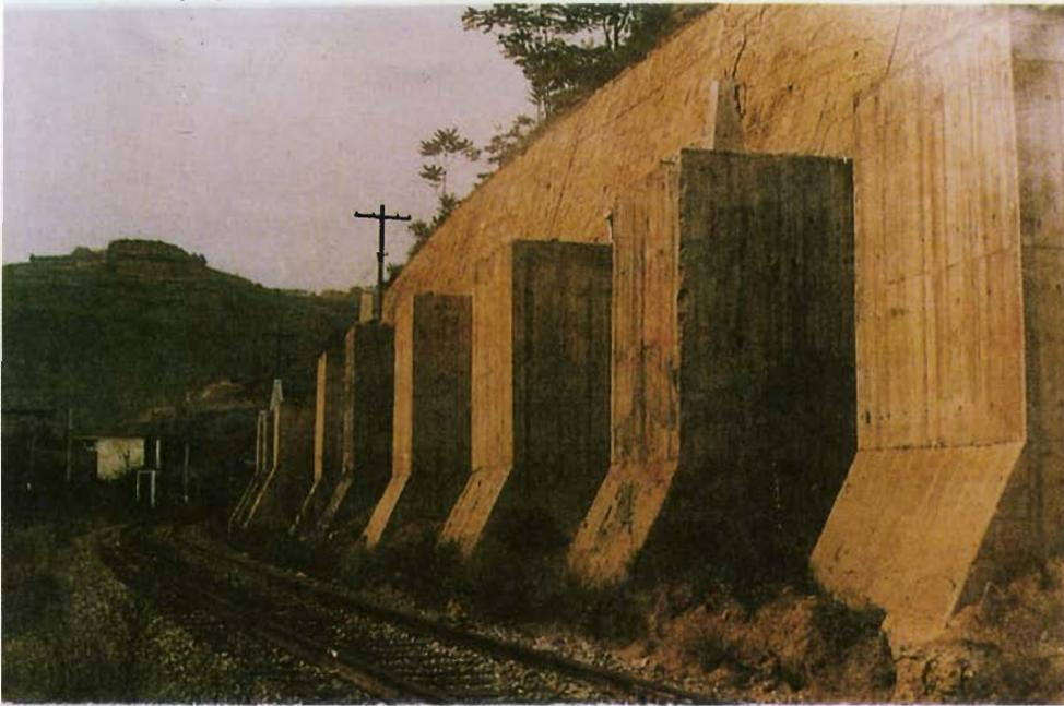
Plate 3: The Use of Skid-Resistant Piles and a Retaining Wall to Stabilise the Landslide, Hangcheng Power Plant, Shaanxi - Ma Shouxin
