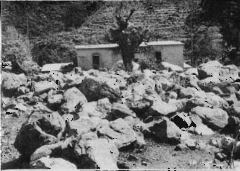
Figure 3: Big Boulders Scattered Downstream of the Breached Landslide Dam
