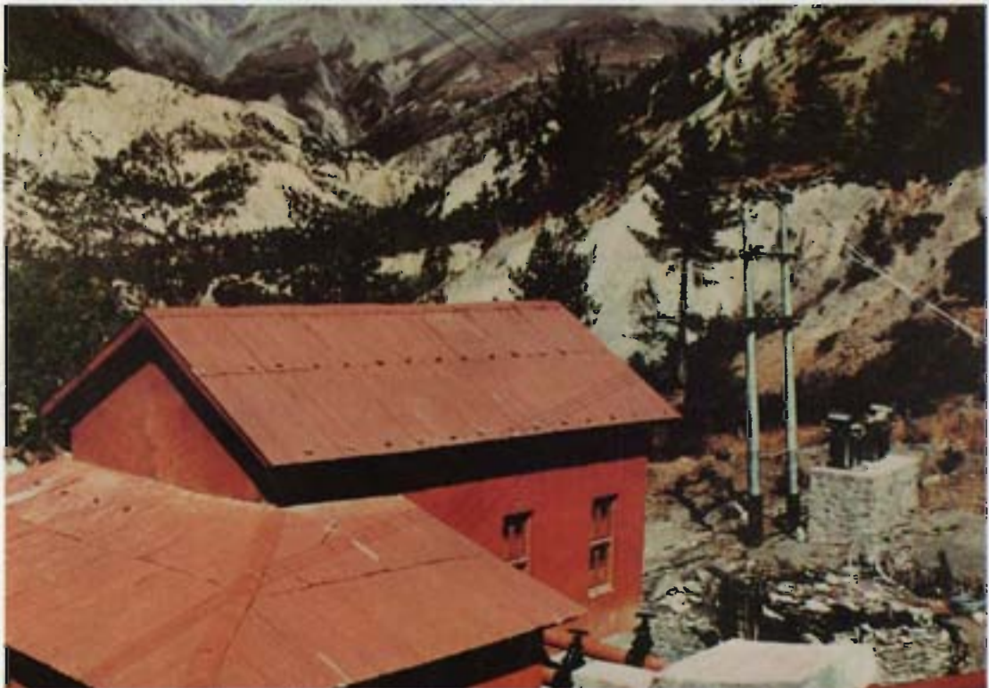
A public sector installation in Manang District which was not operating due to shortcomings in its design and construction.
