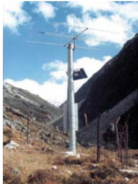
**Figure 6.1:** The transmitter station of Sangma Kharka outside Lake Tsho Rolpa receives signals from sensors and transmits to other remote warning stations.
