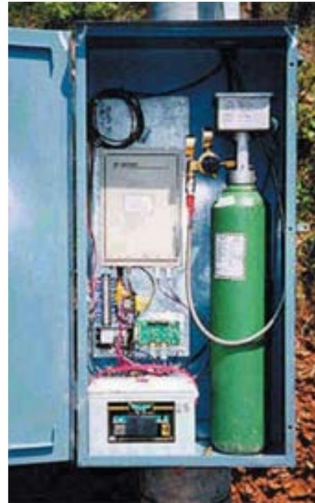
**Figure 6.5:** An MCC 545 unit with 12 V batteries, air cylinder, and MCC-545A RF modem for relay, mounted inside a lockable shelter
