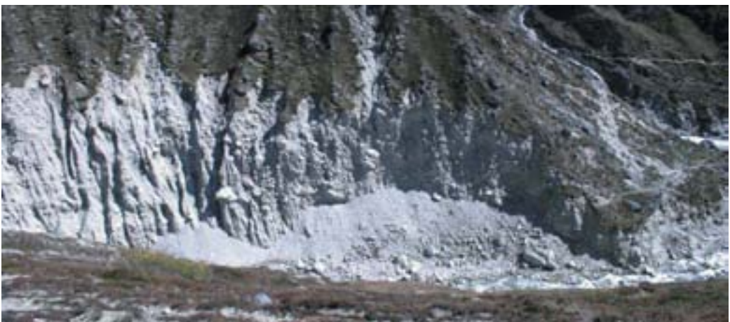
Figure 5.14: Bank erosion at the Bhote Koshi–Langmoche confluence
