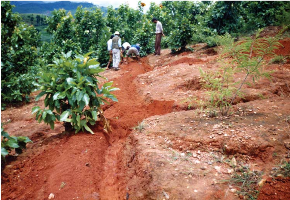
Figure 13.4a: Diversion drains, Nepal
