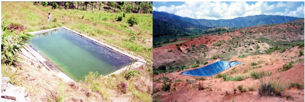
Figure 13.7: Polythene lined water harvesting tanks in (a) Arah rehabilitation site (India) and (b) a rehabilitation site in Nepal
