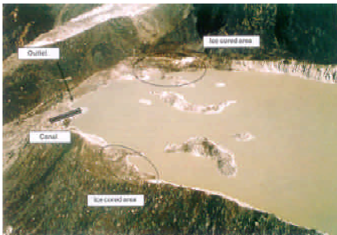
Figure 12.1: Aerial view of end moraine area of Tsho Rolpa Glacial Lake showing the mitigation project construction site (photograph source: DHM 2000)
