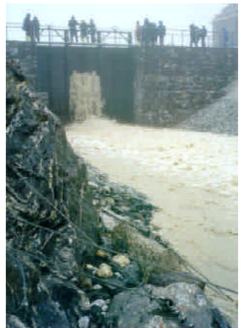
Figure 12.5: Downstream view of outlet canal and gate structure (photo credit: Shrestha 2000)
