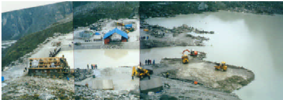
Figure 12.4: Synoptic view of mitigation construction activity at the end moraine of Tsho Rolpa Glacial Lake to reduce the lake water level (photo credit: Shrestha 2000)
