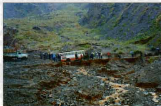
Figure 18.18: The causeway of the highway constructed over the destroyed bridge over the Laogan Ravine. The bridge was damaged by a debris flow in May 1990
