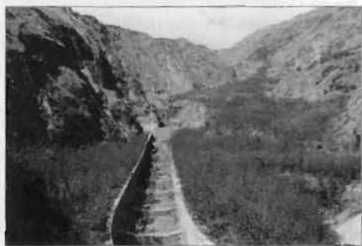
Figure 18.21: View of channelised ravine course (diversion flume), with scour-proof ribs and fixed-bed dams, and of bio-engineering structures in the valley of the Laogan Ravine
