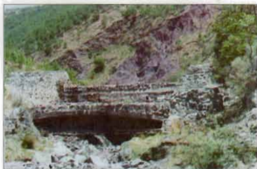
Figure 18.6: Sediment trapping dam with single-arch foundation constructed across the main stream of the Heisha Ravine
