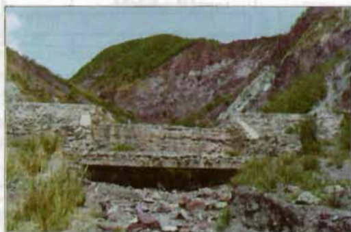
Figure 18.7: Sediment trapping dam with plate foundation constructed in the landslide area of the mainstream of the Heisha Ravine
