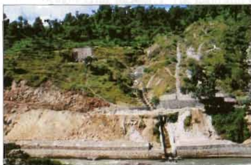
Figure 17.29: Landslide AH-4: landslide drainage and bank protection upstream from the landslide
