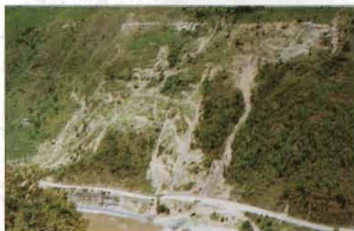
Figure 17.25: Landslide AH-1: a complex network of landslide drainage
