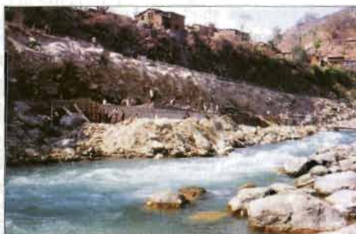
Figure 17.30: Landslide AH-4: construction of revetment wall
