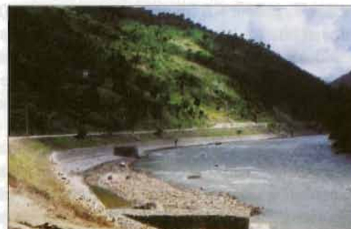
Figure 17.28: Landslide AH-1: completed bank protection works
