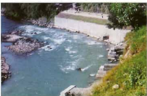
Figure 17.31: Landslide AH-4: completed revetment wall
