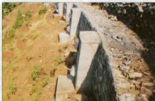
Figure 17.26: Landslide AH-1: an anchored gabion-retaining structure
