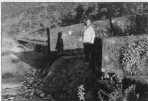
Figure 15.6: Displacement of the drainage masonry wall at the toe of the slope
