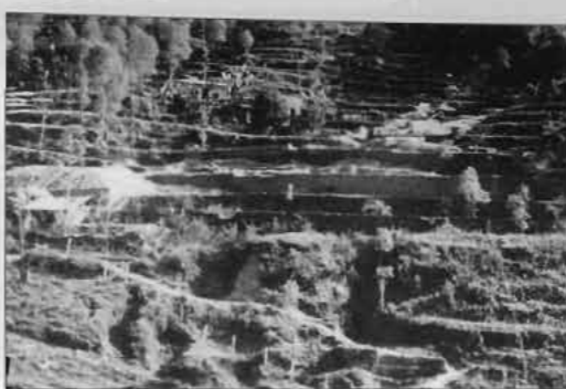
Figure 15.5: Debris accumulation at the check dams brought down by the debris torrent of July 1995
