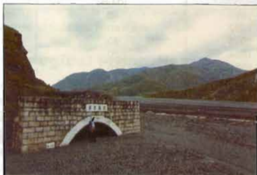
Figure 13.5: A tunnel along the Dongchuan railway line was silted up by debris flow in
