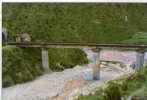
Figure 13.6: Central pier of a railway bridge damaged by a debris flow, Dongchuan, Yunnan
