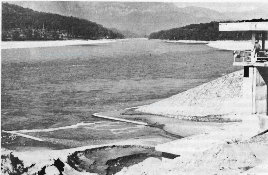
Photo XIV - Narayanghat, Chitwan District - Irrigation intake on Narayani River completely choked with sediment. A better design could have significantly reduced this sedimentation.
