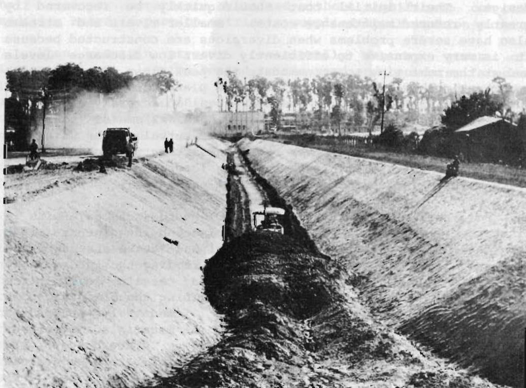
Photo XV Narayanghat, Chitwan District - Sediment removal from the main canal, Chitwan Irrigation Project. Over 2.5 meters of fine sand were deposited in this canal during the 1984 monsoon, completely blocking irrigation water flow. Better use of available data could have warned designers of such a hazard.
