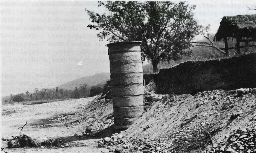
PHOTO XVII - Near Waebater Village, Marin Khola, Sindhuli District. River scouring has exposed 6 rings of this concrete lined well, leaving behind a monument to the fury of the Marin Khola in flood. Throughout the watershed, many river banks were eroded destroying many hectares of farmland.
