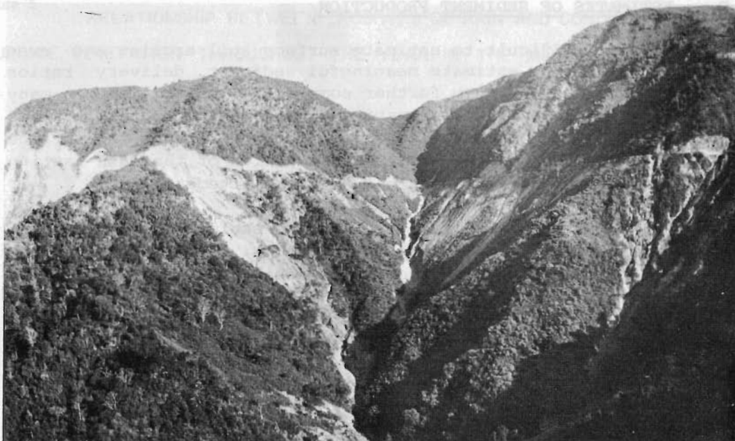
PHOTO V. - Feeder road construction northeast of Dharan. Severe erosion has been initiated by the poor layout, design and construction technique of this road. This alignment has since been abandoned as too costly to construct and maintain.
