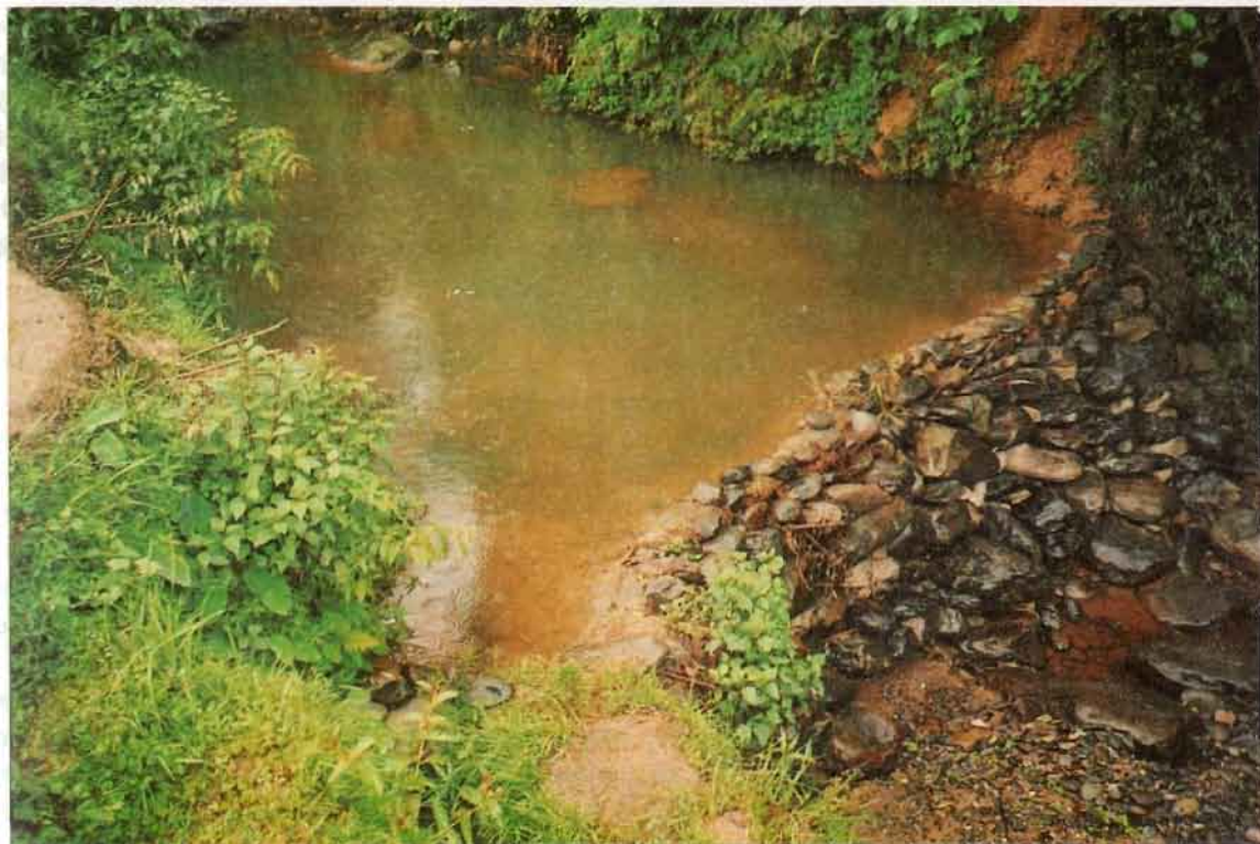
Figure 6. Typical diversion dam used for irrigation in the Andheri Khola sub-watershed.
