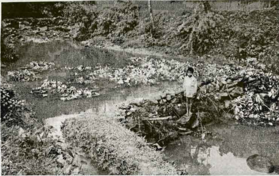
Figure 2. Diversion dam in the lower reaches of the Andheri Khola.
