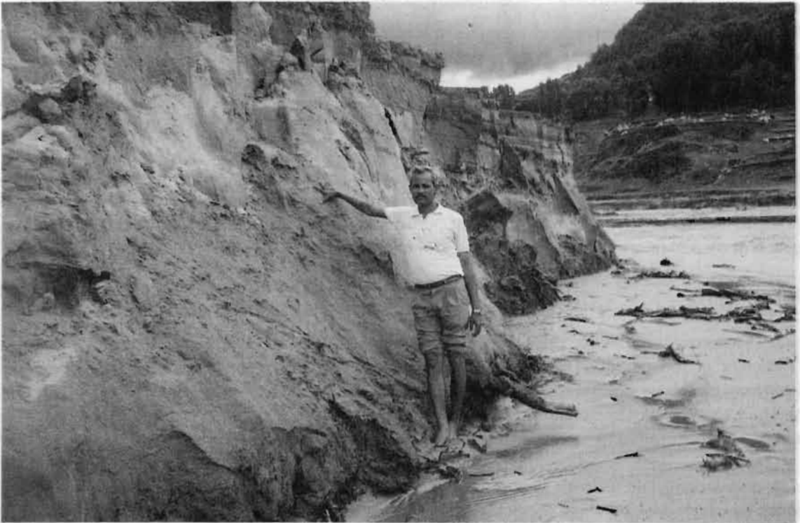
Figure 9. Kulekhani Reservoir Delta. Headcutting of sand and gravel deposit during low stages of the reservoir. The deposits are primarily sand with gravel lenses near the top (June, 1994).
