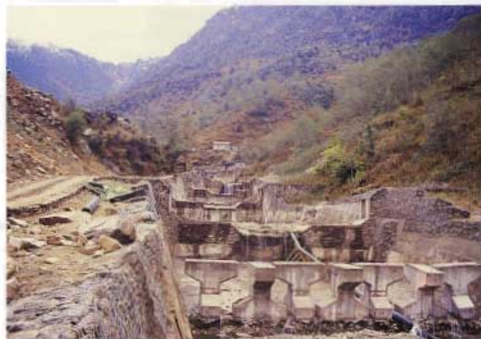
Prevention of bed scour and bank sliding of a steep mountain stream, with thick (more than 30 m) soil cover, by use of concrete armour blocks (tetrapods), along the Charnawati River, Nepal.
