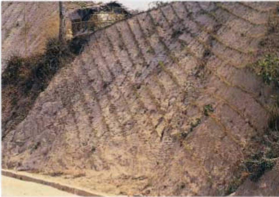
Diagonal grass lines planted on a steep slope
