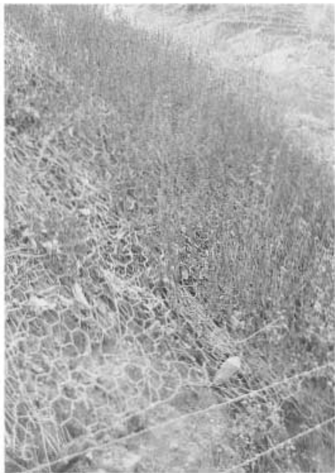
Covering the ground with salvaged gabion net has helped revegetation.
