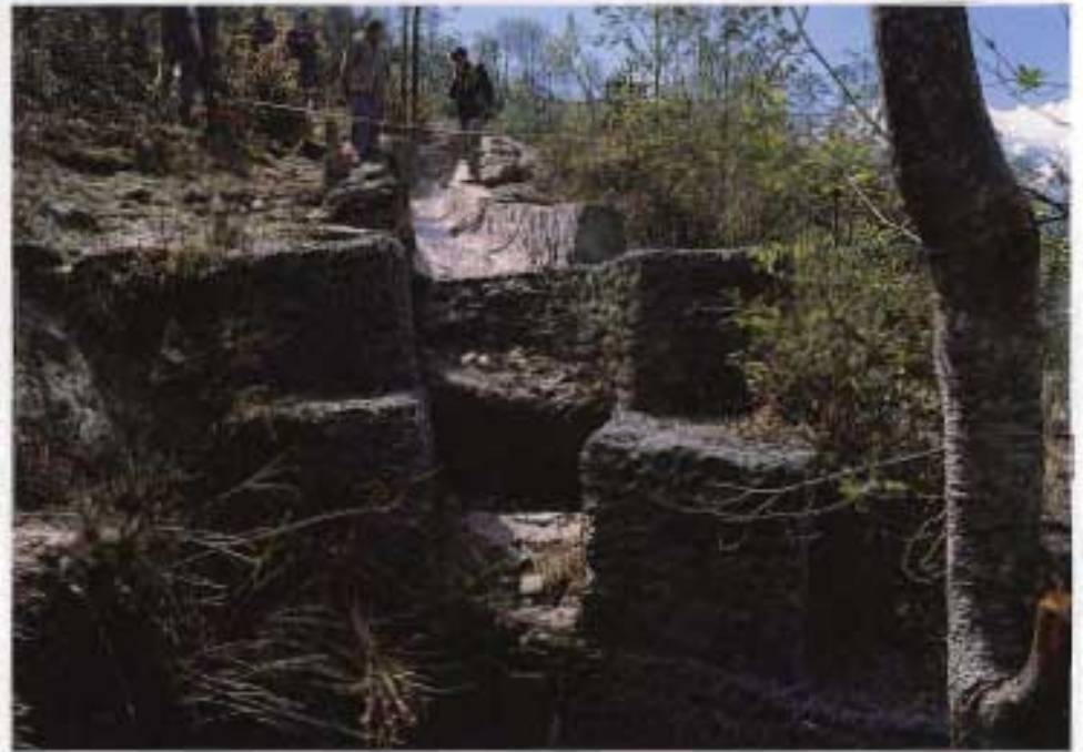
A cascade for gully control
