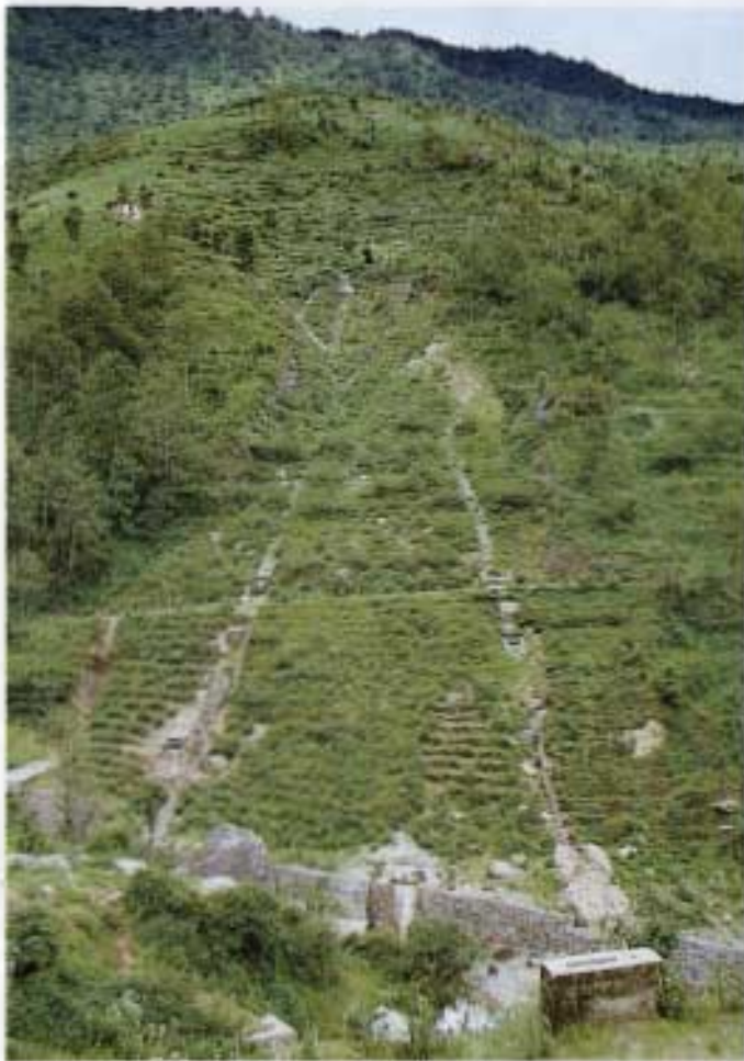
A combination of biotechnical and landslide drainage measures stabilize a landslide that damaged the road. The photograph on the left shows the completed works, while the photograph to the right shows the same site under construction.
