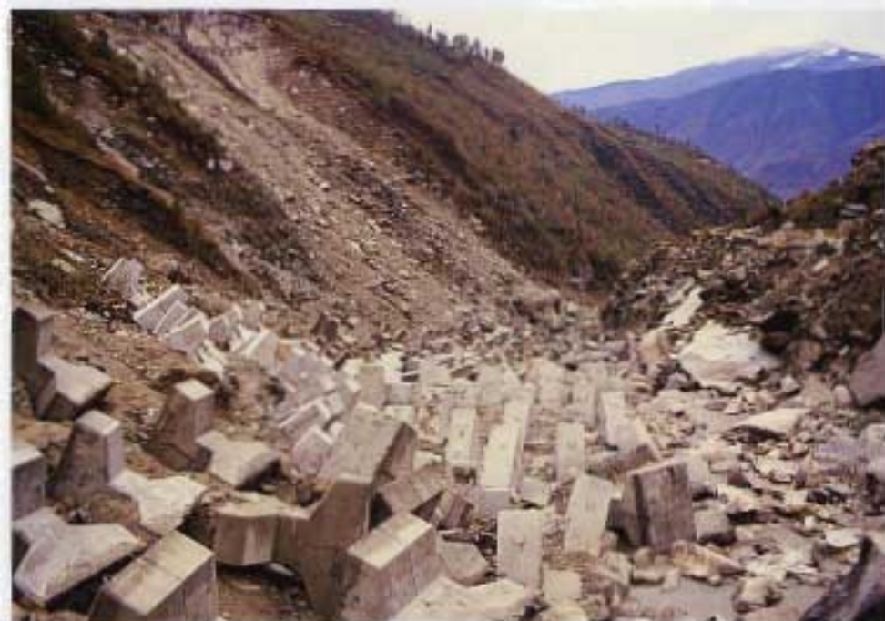
Prevention of bed scour and bank sliding of a steep mountain stream, with thick (more than 30 m) soil cover, by use of concrete armour blocks (tetrapods), along the Charnawati River, Nepal.
