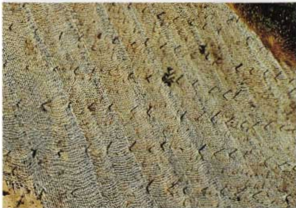
Cuttings are fixed with stake and covered by jute net manually.
