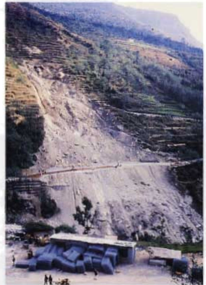
A combination of biotechnical and landslide drainage measures stabilize a landslide that damaged the road. The photograph on the left shows the completed works, while the photograph to the right shows the same site under construction.
