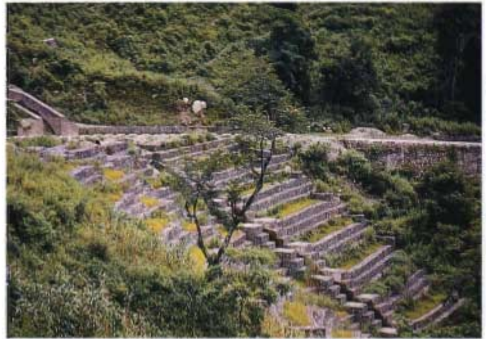
Terracing of slope below road and grass planting
