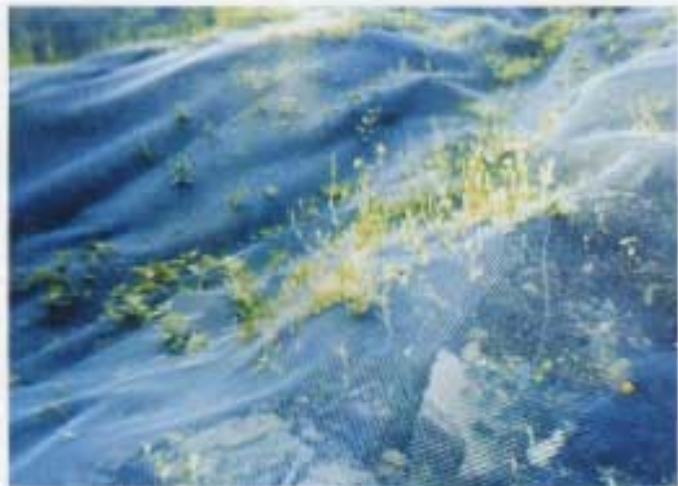
Cuttings fixed and covered by synthetic fabrics
