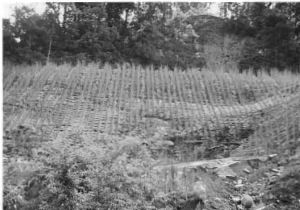
Downslope grass lines planted on the poorly drained Siwalik mudstone.
