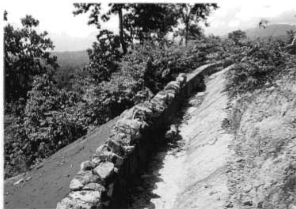
A lined catch drain above the cut slope
