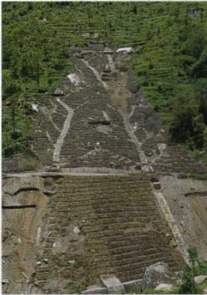
Landslide stabilized by a sub-surface drainage network
