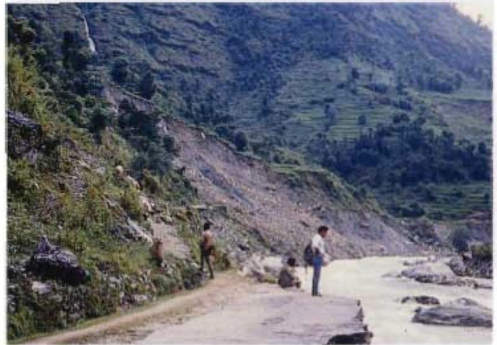
A complete washout of the road by the river
