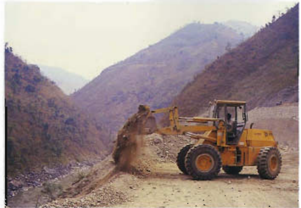
Side casting during construction
