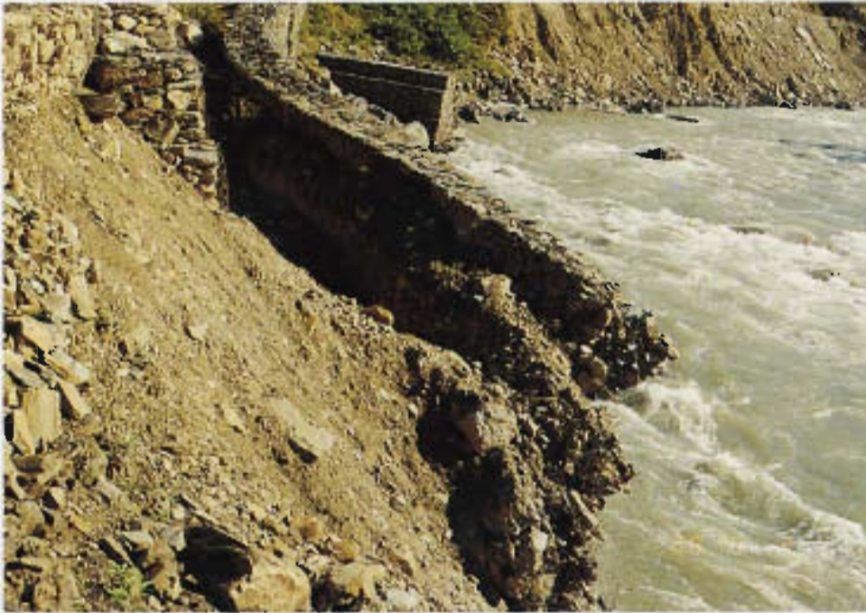
Gabion spur failures, first by scour and then by rupture of wires
