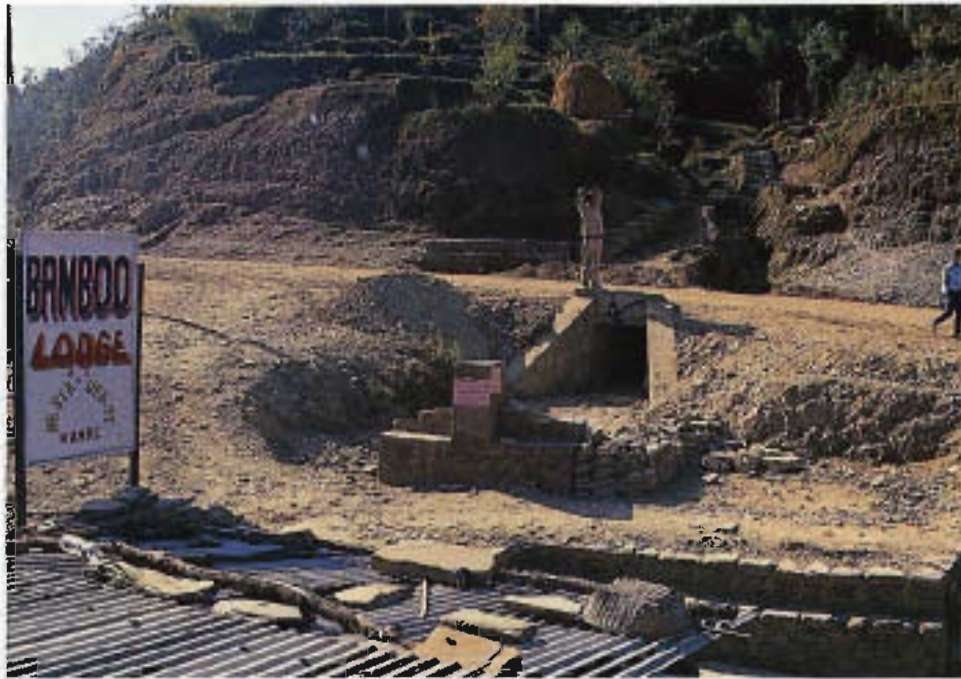
A culvert outlet is directed towards an existing building, flooding the latter.
