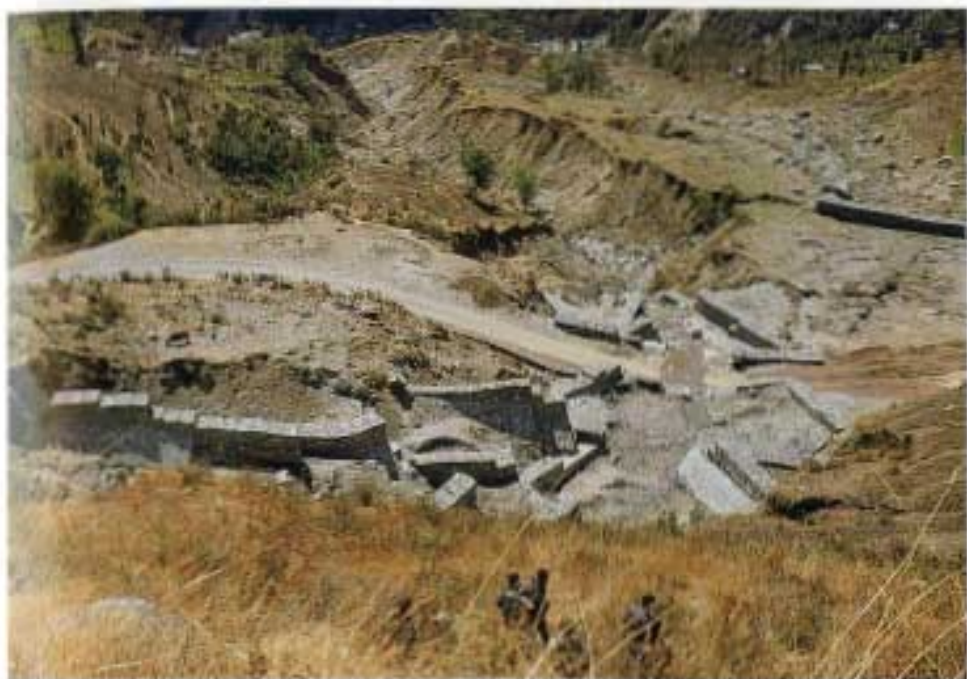
Massive gullying after heavy rainfall in this more than 50m deep colluvium/till washed out several houses, killing their occupants, in 1987; the Lamosangu-Jiri Road, Nepal.
