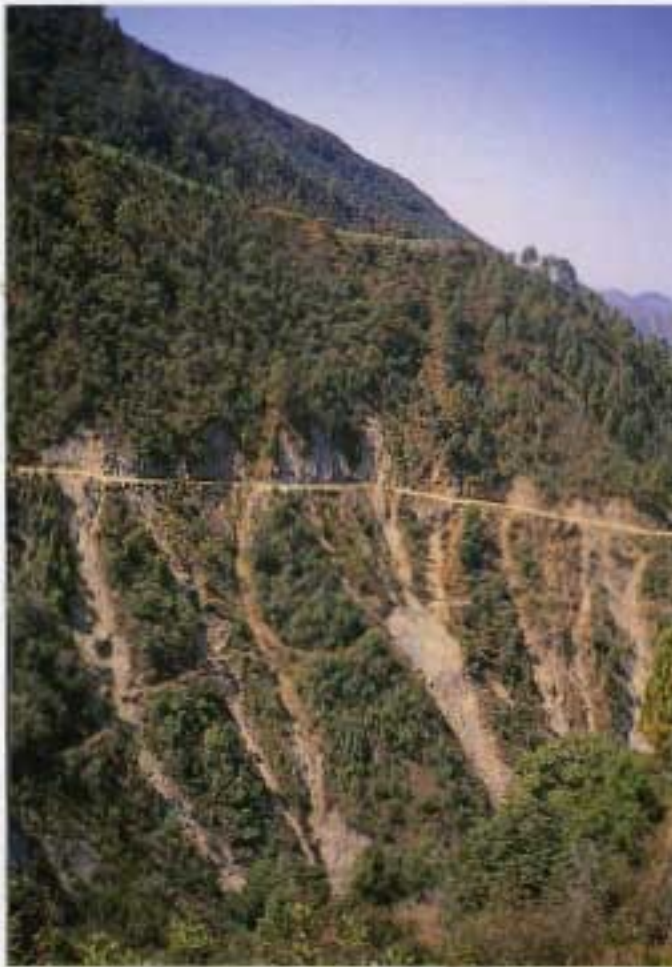
Devegetation and scars from indiscriminate side casting
