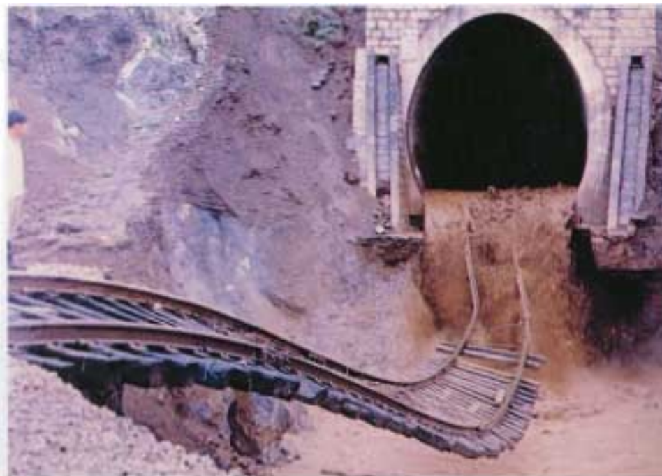
Massive damage to railway track by a large-scale debris flow in China
