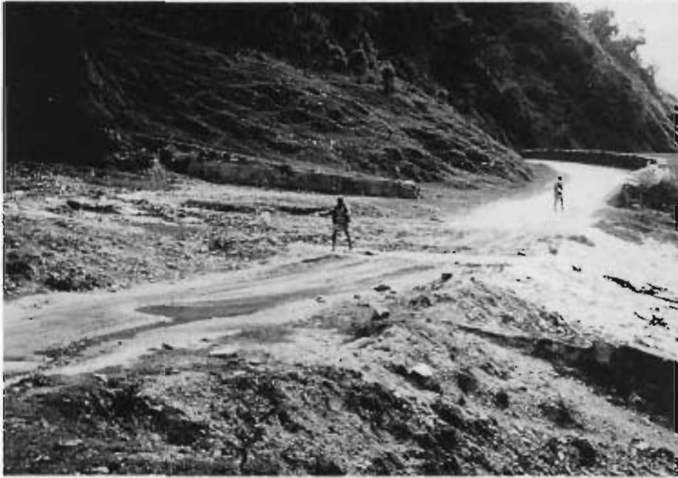
A large culvert (right) and causeway (left) on a valley road
