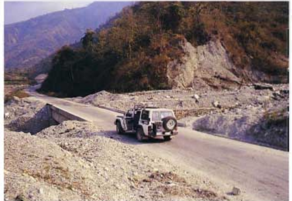
Severe undercutting problems exist in valley roads crossing young streams.
