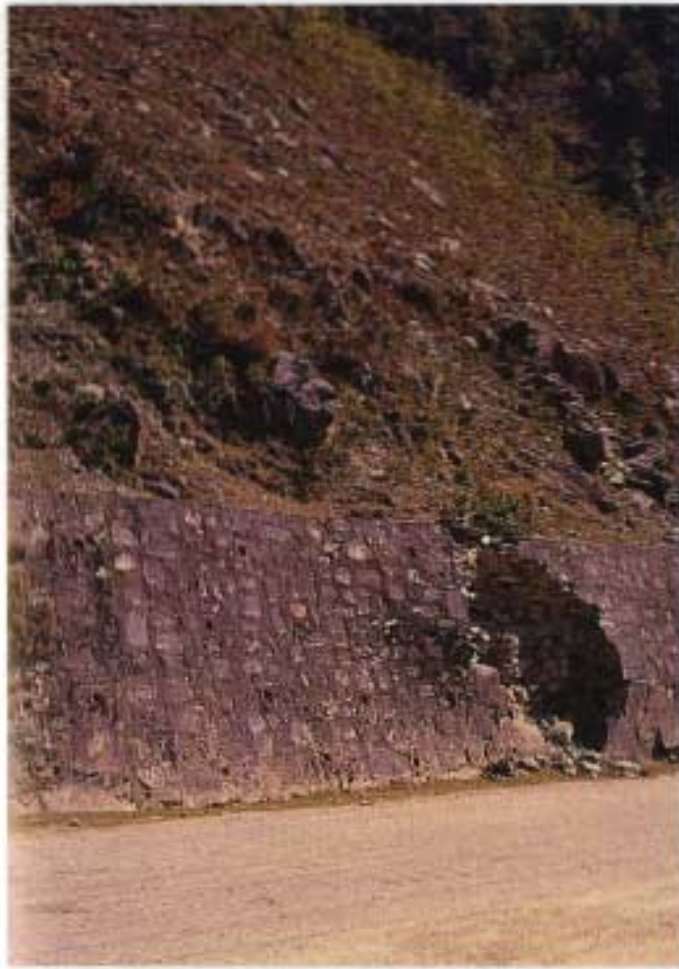
▲ Breast wall failure from hydrostatic pressure
