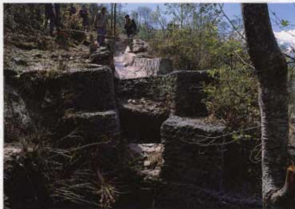
A cascade for gully control
