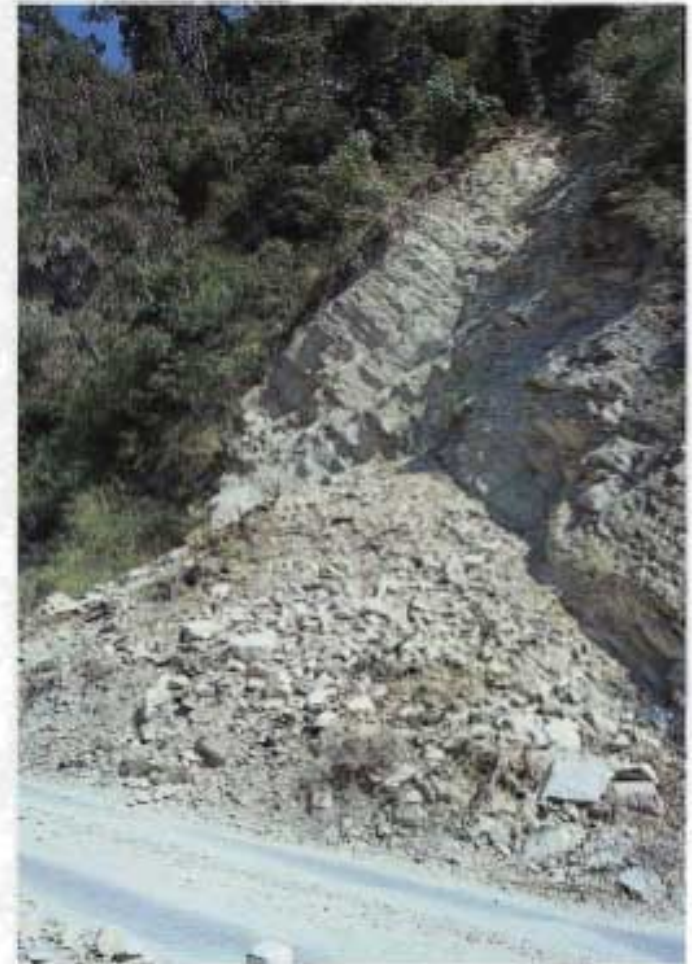
A wedge failure in the weathered rock. Three sets of joints are visible.
