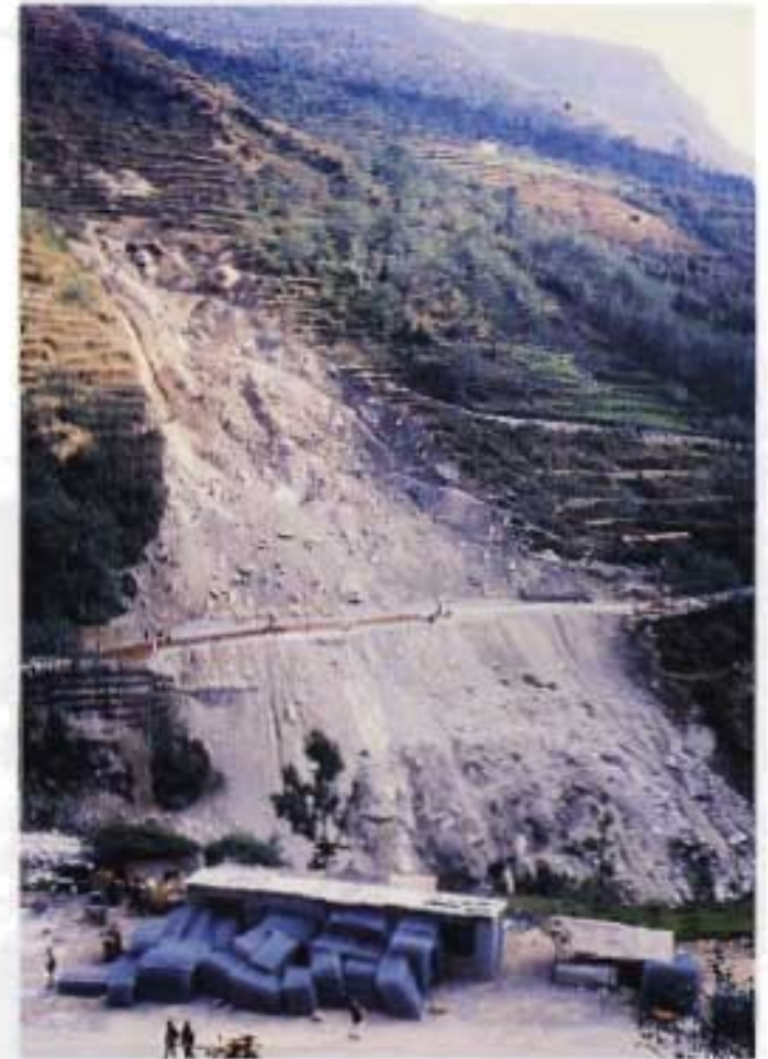
A combination of biotechnical and landslide drainage measures stabilize a landslide that damaged the road. The photograph on the left shows the completed works, while the photograph to the right shows the same site under construction.
