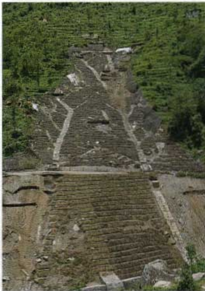
Landslide stabilized by a sub-surface drainage network
