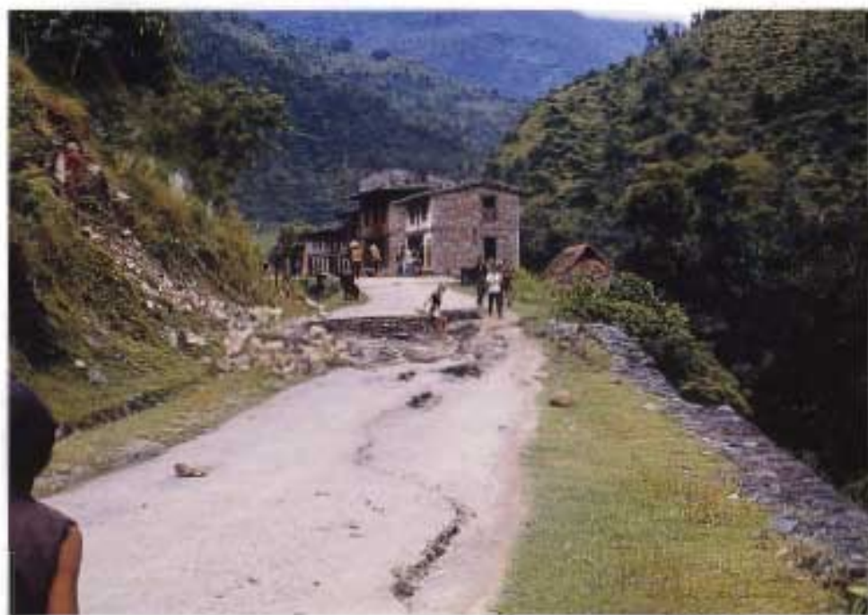
A deep seated rotational slide damages the road.
