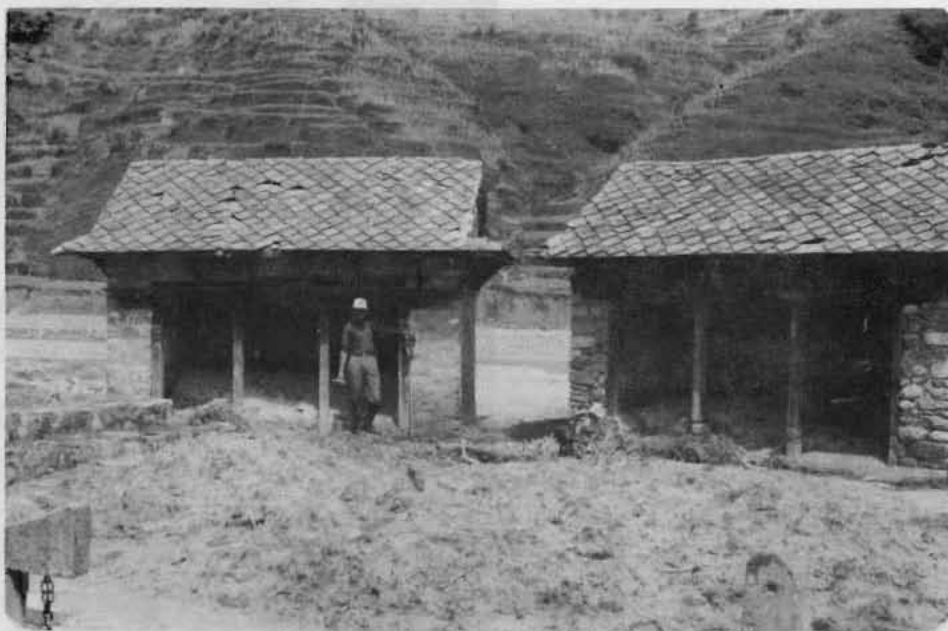
Plate 46: The sand and silt deposits in the temples at Indrenithan, about 70 cm above ground level. View towards the west
