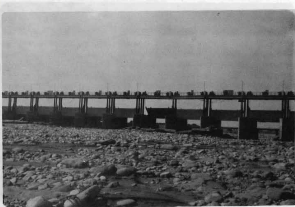
Plate 55: Downstream view of the Bagmati Barrage and the mid-channel bar. Notice a damaged gate (in the centre) and a 33 m long tree trunk. The Bagmati Bridge is seen in the background. View towards the south
