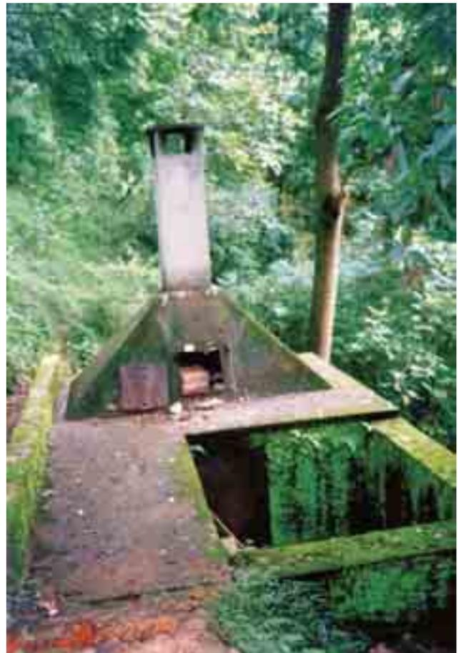
Abandoned Chamber Built for Burning Medical Waste
