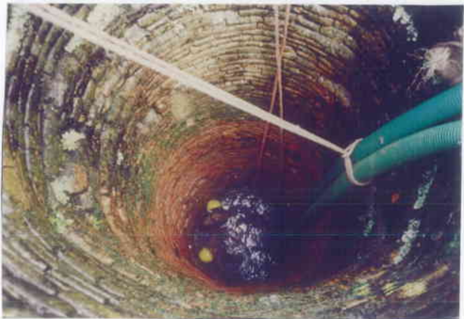
Plate 6 : Deteriorating Condition of a Dug Well in Urban Patan
