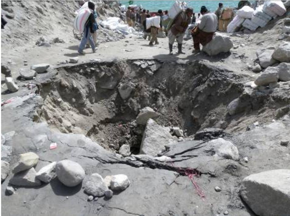
Figure 14: Sinkhole formed on 14 April 2010 on the dam, from the lake side.
