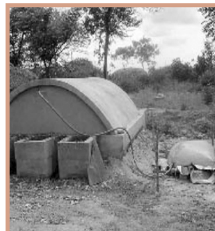
An 8 m 3 biomass based biogas plant under commissioning trials, operated largely with parthenium as the main feed. A larger biogas bag was used to store the biogas produced and when needed to be transmitted to houses, a weight was placed on the bag to increase the line gas pressure. This plant could not be operated for long due to a shortage of biomass at the village. (Photo courtesy Dr. Chanakya)
