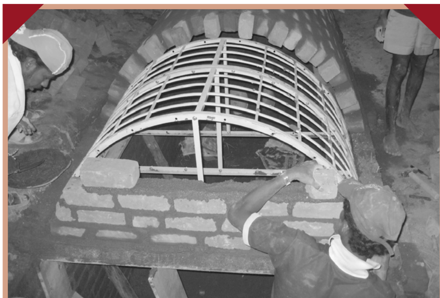
Construction of a 3B masonry vault with collapsible mould (Photo courtesy Dr. Chanakya)
