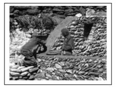
Mud bricks or rammed earth provide good insulation. If mud is not available, walls can also be built in stones. South wall measures 3,5 ft and North one 7 ft.
