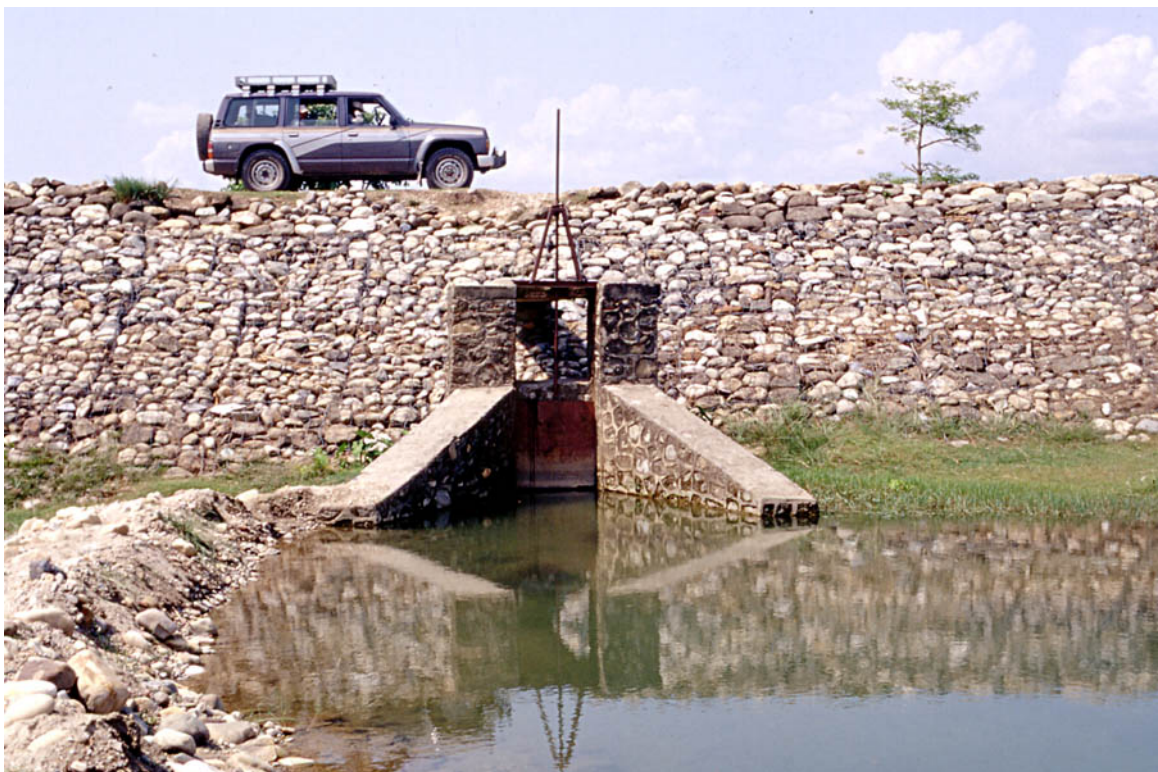
Plate 10: River training structure on the right bank of Rapti River to reduce flood hazard and one of the intakes of irrigation canal.
