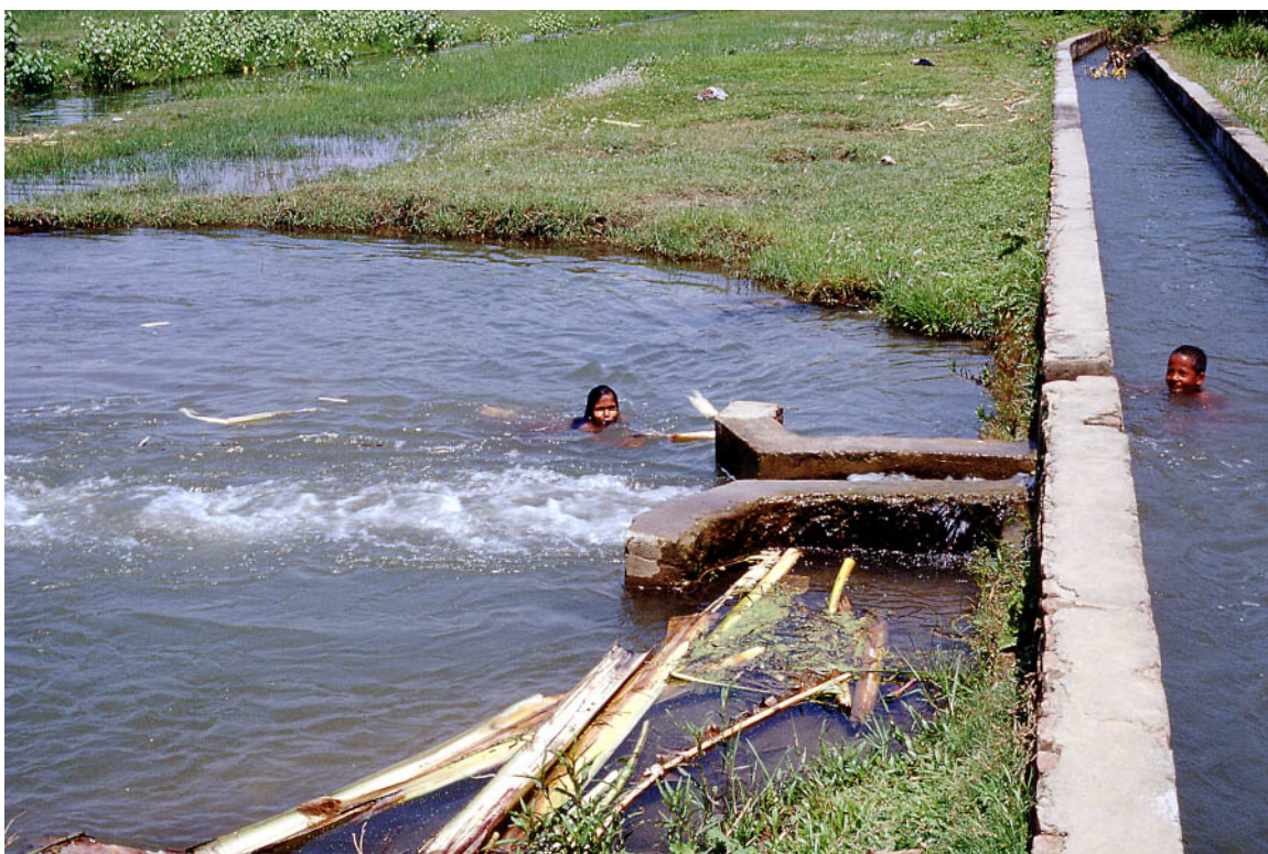
Plate 08: Distribution channel to irrigate the agricultural field.
