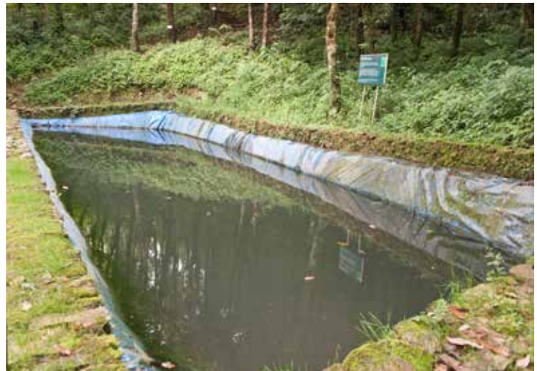
Water harvesting pond
