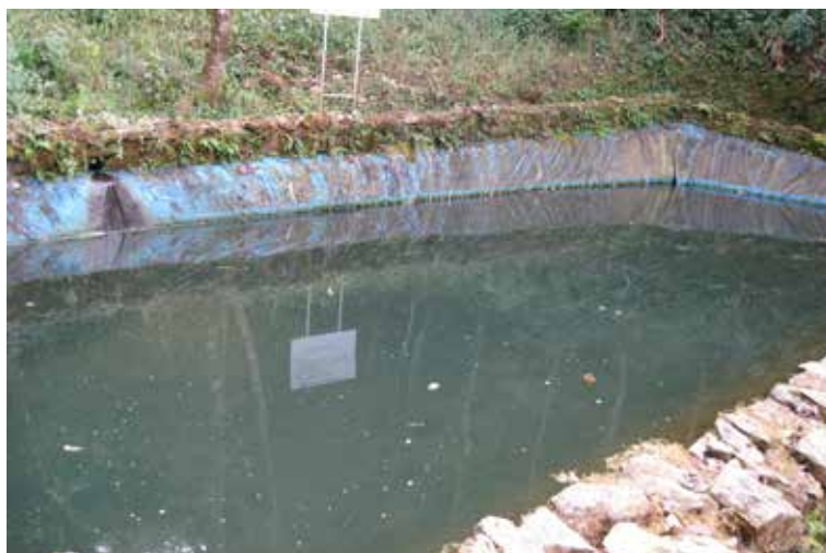
Water harvesting pond
