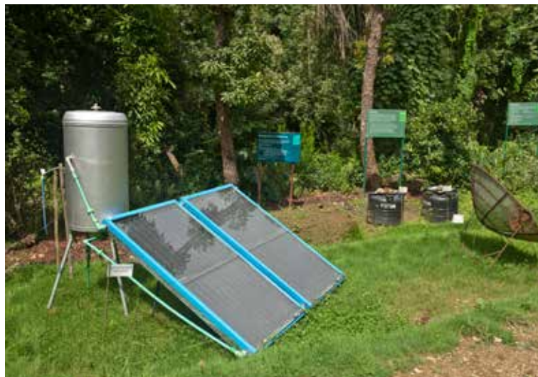
Solar water heater
