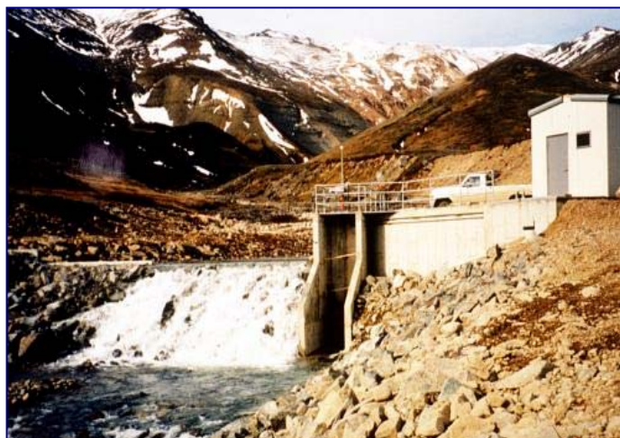
This small scale hydro system can provide power for a community of 800 people. (Photo courtesy Warren Gretz and NREL).
