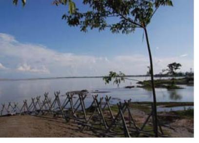
Figure 22: Away from us! Holding back the river with porcupine anti-erosion measures at the breached portion (eastern) of the Matmora embankment
