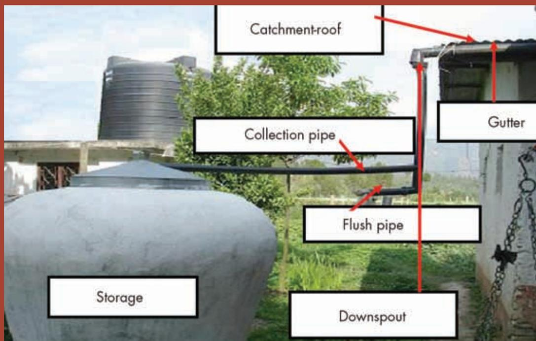
at the inlet of the storage to avoid the entry of insects. For irrigation purposes, pre-filter to keep out sediment build-up if the sediments cannot be easily removed from the storage sub-system. Sedimentation chambers before the storage can be made to filter sediments entering the storage.
