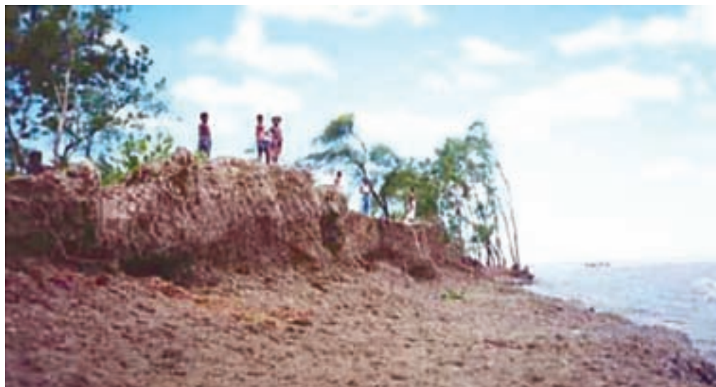
Figure 3: River bank erosion
